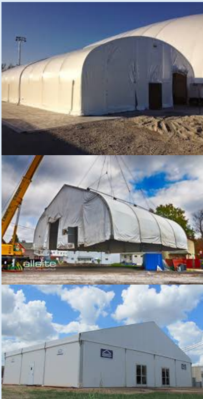
Figure 1. A temporary structure will be constructed over Zone A to eliminate potential emissions from the work activities. See A1 for more details.
