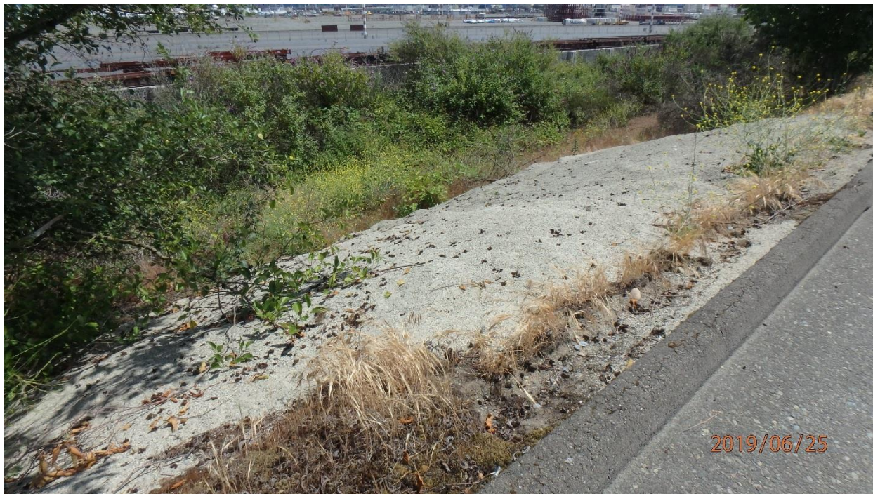
Photo 7. Representative photo of two areas on east landfill slope, cleared of vegetation and covered with loose sandy soil: RA-3 (map notes 8 and 9)
