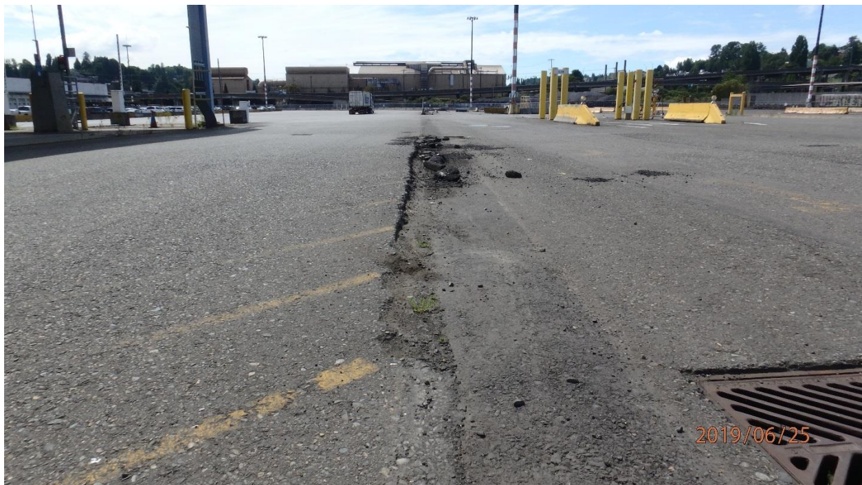
Photo 6. Pavement deterioration: RA-2 (map note 6)
