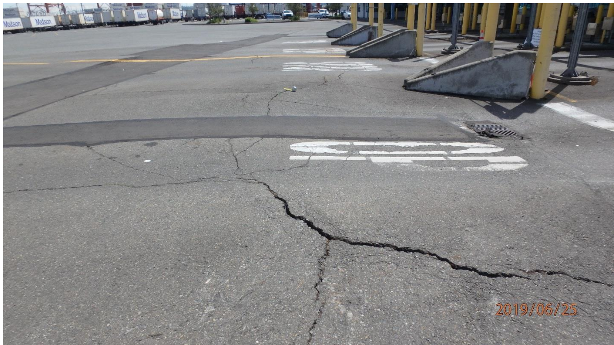
Photo 4. Mound in pavement with cracks as wide as 2 in.: RA-2 (map note 5)
