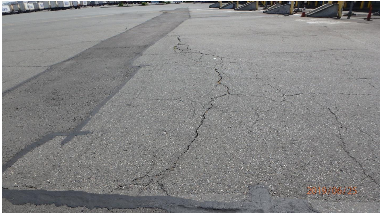
Photo 2. Elongated mound in pavement with cracks as wide as 1 in.: RA-2 (map note 4)
