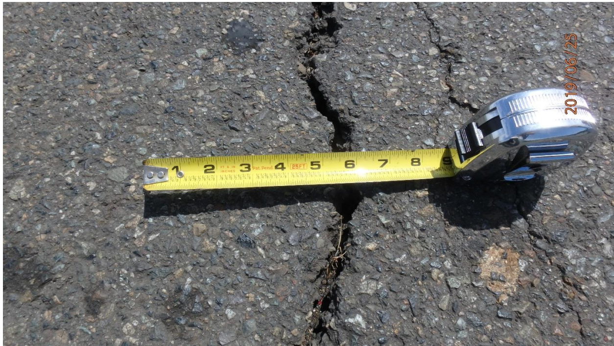
Photo 3. Close up of elongated mound in pavement with cracks as wide as 1 in.: RA-2 (map note 4)
