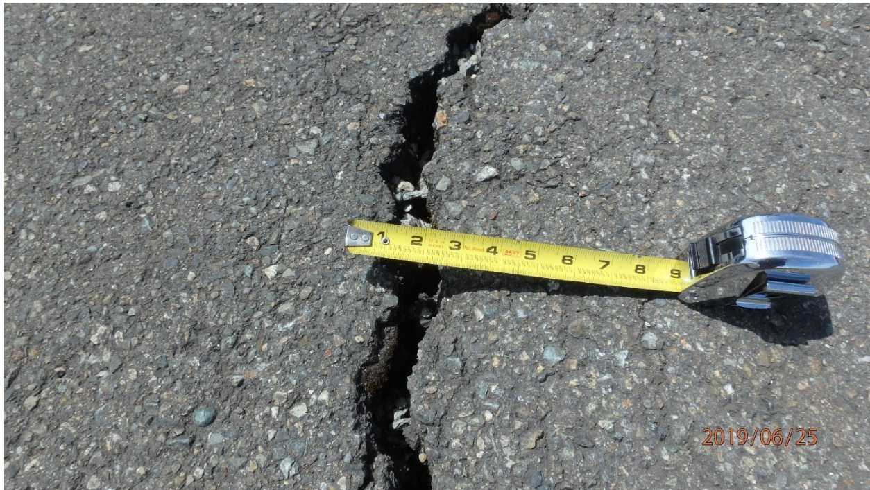
Photo 5. Close-up of mound in pavement with cracks as wide as 2 in.: RA-2 (map note 5)
