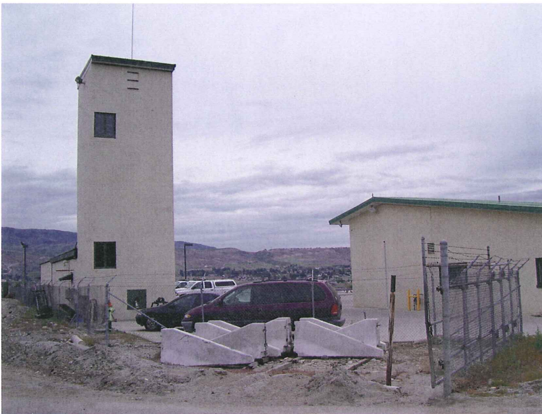
Northwest corner of Fire District property
