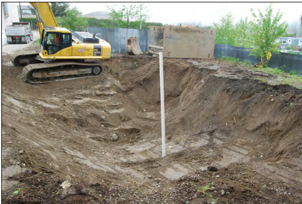
Photograph 12: May 17, 2011 - View northeast across the excavation as backfill proceeds.
