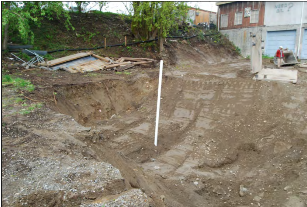
Photograph 11: May 17, 2011 - Looking southwest across the excavation as it is being backfilled.
