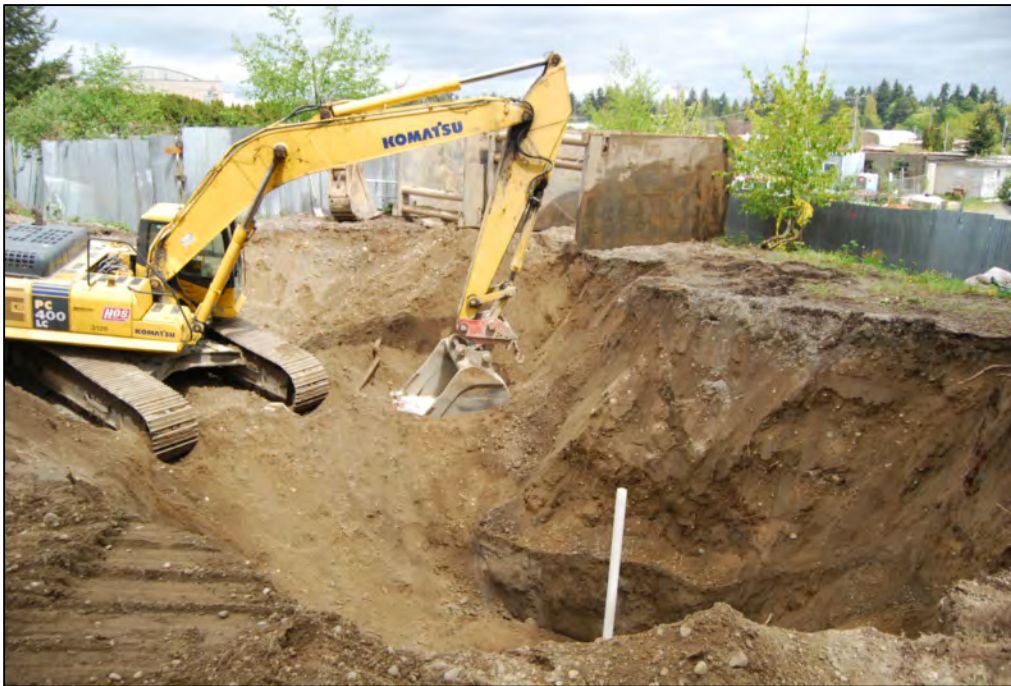
Photograph 10: May 16, 2011 - Looking northeast during the backfilling with in-situ overburden.
