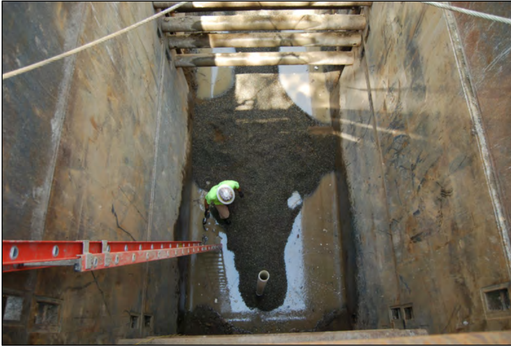
Photograph 7: May 13, 2011 - Vertical riser has been placed on the groundwater remediation system.
