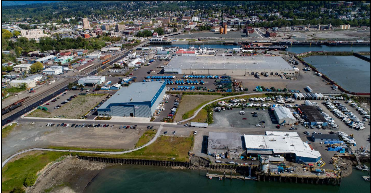
Figure 4: Central Waterfront site with completed All American Marine building, May 2019
