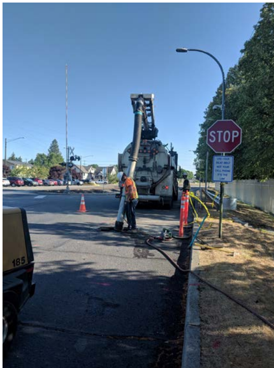
Able Cleanup Technologies air knifing monitoring well MW-1A. (view looking north)
