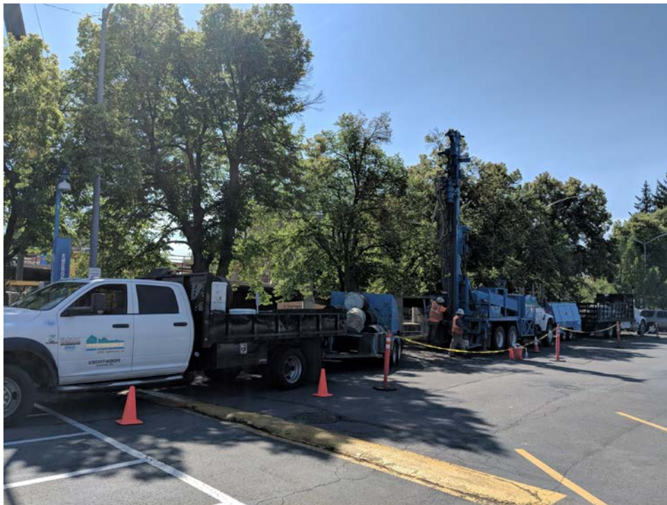
Environmental West Exploration Drilling installing MW-5B using air rotary drilling.
