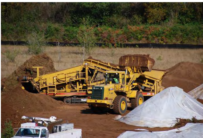
Close-up view of screening operations
