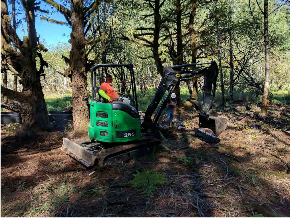
Installing Silt Fence, RAU 2A-16
