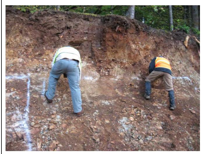
Identifying step-outs for further excavation on berm
