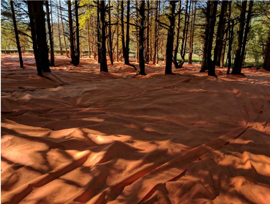
Installing demarcation geotextile, RAU 2A-16
