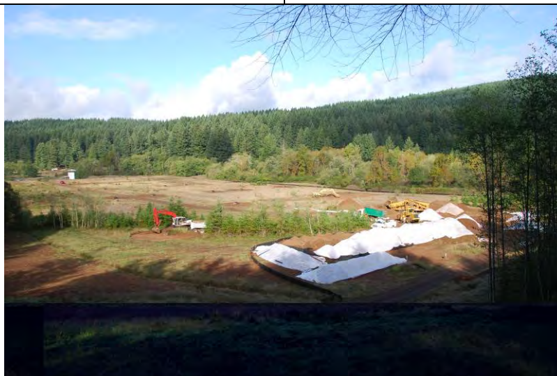
Panoramic view of operations within range floor areas
