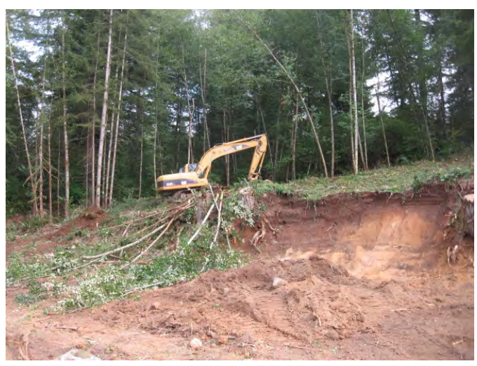
Excavating range floor areas uphill of berm
