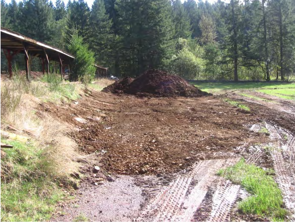
Loading Soil for Disposal, October 2010
