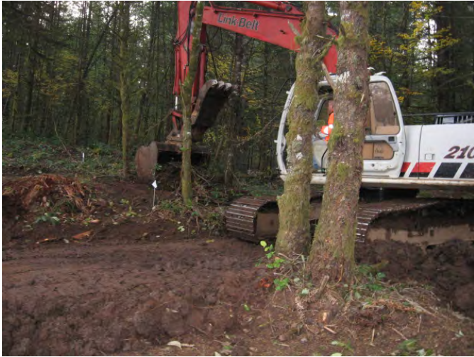
Excavating range floor
