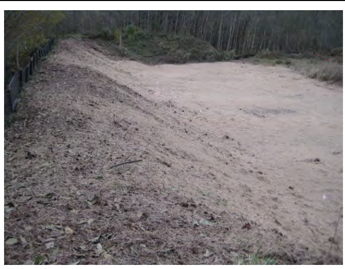
Erosion mulching completed on berm and range floor
