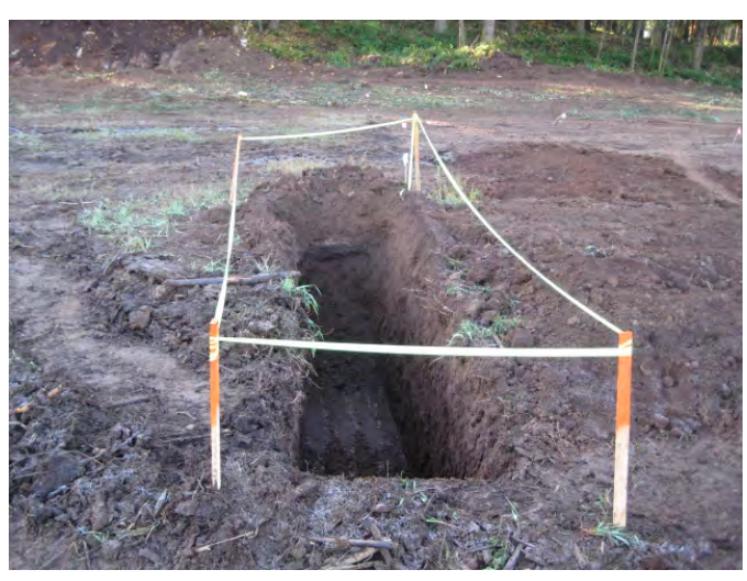
Investigative trenches on range floor
