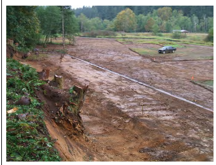
Completed first round of range floor excavation
