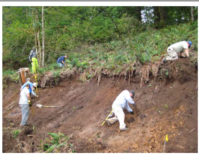
MEC clearance being performed prior to excavation
