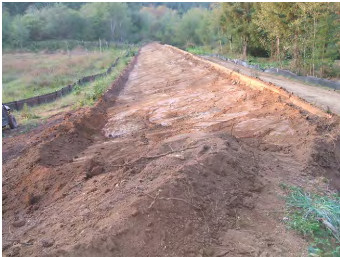
Face of berm after first round of excavation
