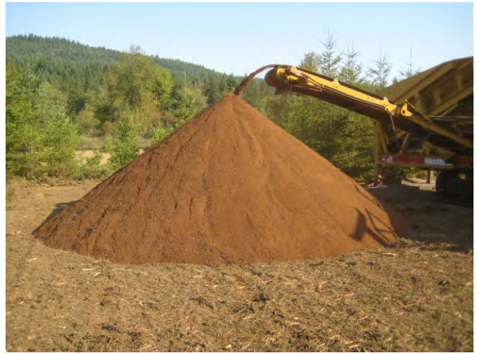
Screened product (fines < 0.5 inches in diameter)
