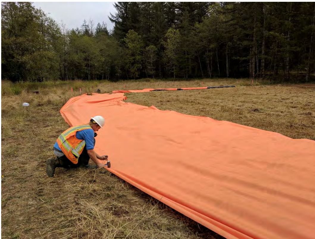
Installing demarcation geotextile, RAU 2A-21
