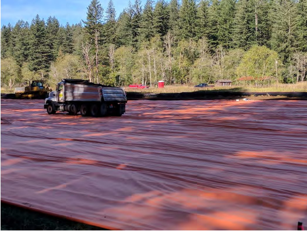
Placement of 1-foot soil cap over demarcation geotextile, RAU 2A-21
