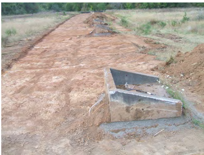
Excavation around pop-up target bases on range floor
