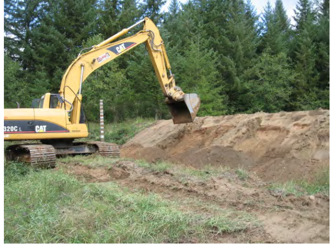
Excavating front face of berm
