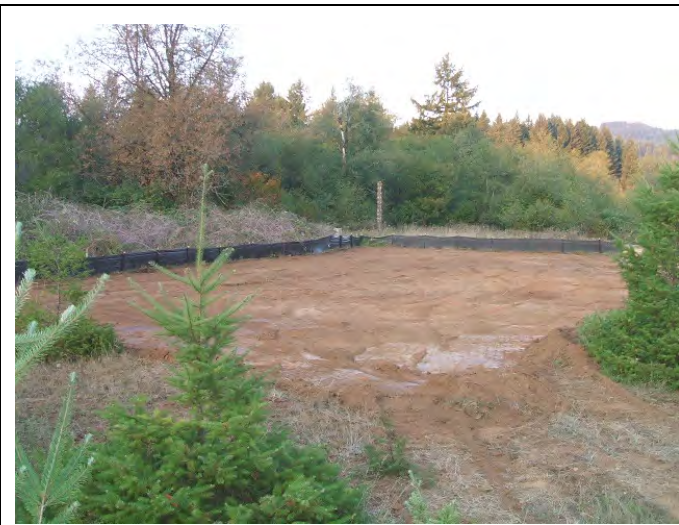
Excavation on range floor areas
