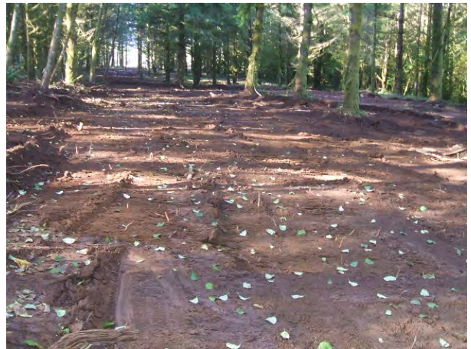
Excavation on range floor areas
