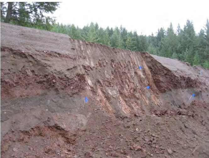
Step-outs being cut on the berm face
