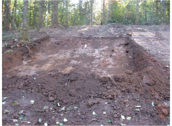
Excavating step-outs on range floor
