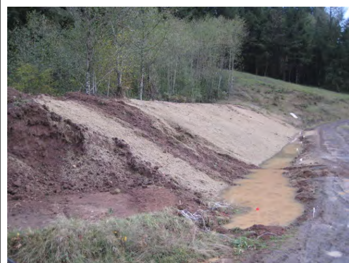
Erosion mulching completed on the berm face
