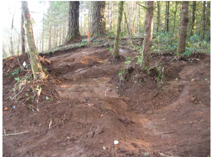
Excavating step-outs on range floor
