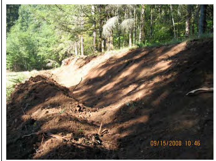
Exposed berm face after first round of excavation
