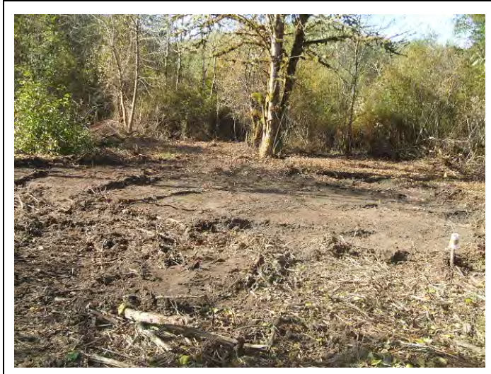
Excavation on range floor areas
