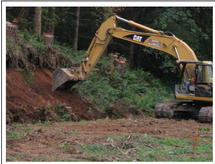
First cut on the Westside of berm face
