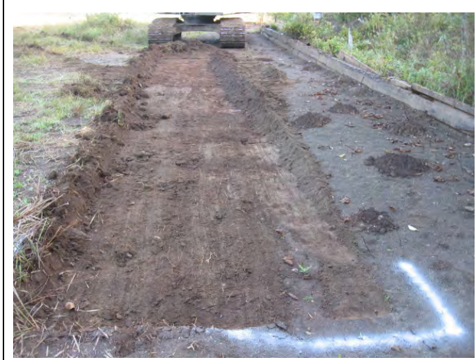
Step-outs being cut on the berm face
