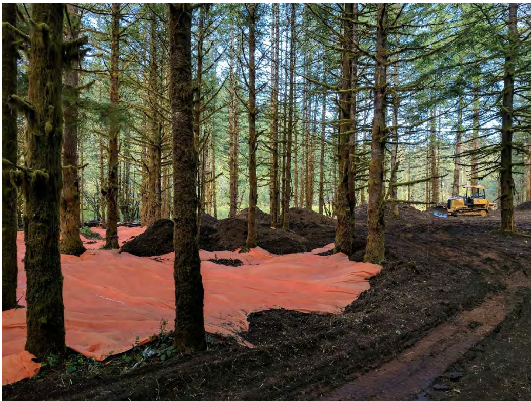
Placement of 1-foot soil cap over demarcation geotextile, RAU 2A-16
