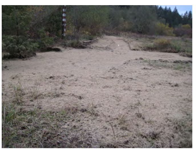
Erosion mulching completed at the range
