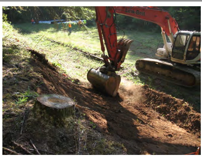
Excavating berm face
