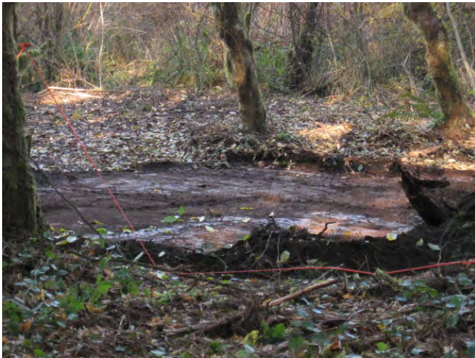
Excavating range floor
