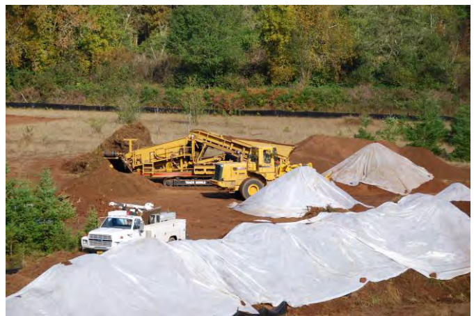
Soil piles staged after screening pending treatment
