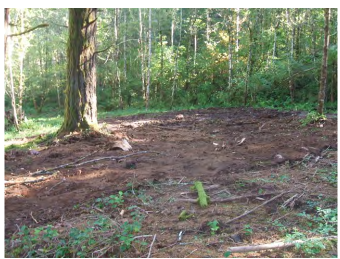
Excavation on range floor areas
