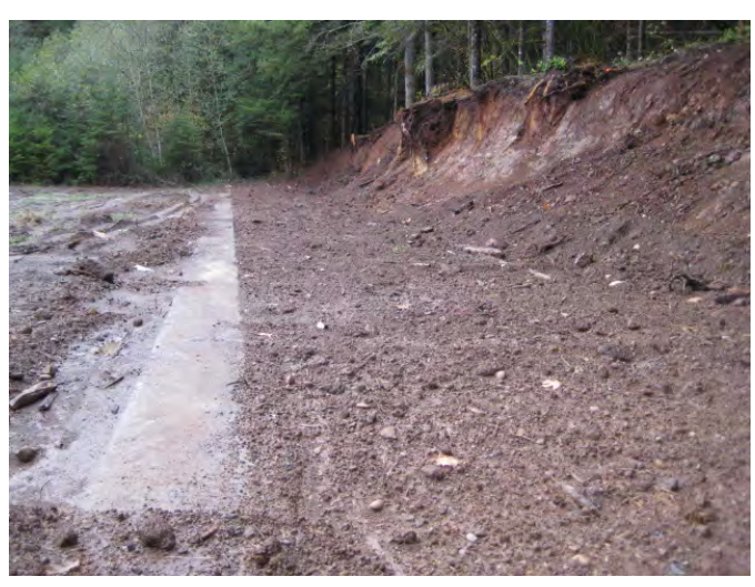
Back-filling completed at toe of berm
