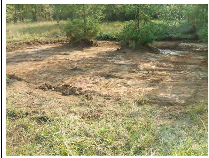
Completed range floor excavation on range floor
