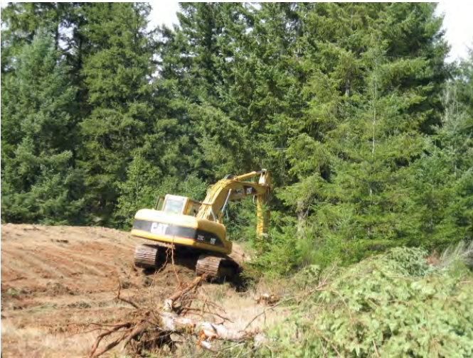
Excavating on back-side of berm face
