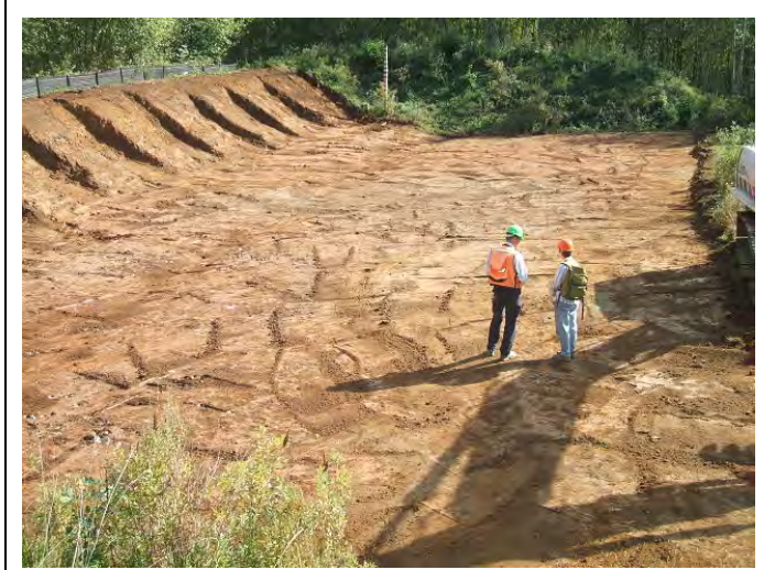
Archeological investigation on berm face and range floor
