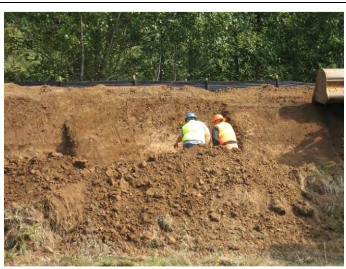
Excavating front face of berm
