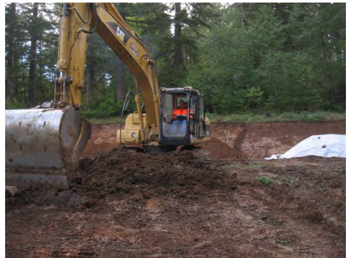
Excavating rang floor around pop-up targets
