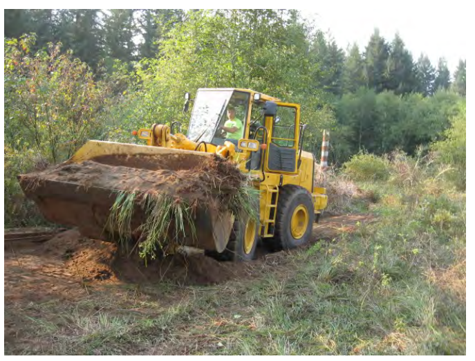
Hauling soil excavated from berm face
