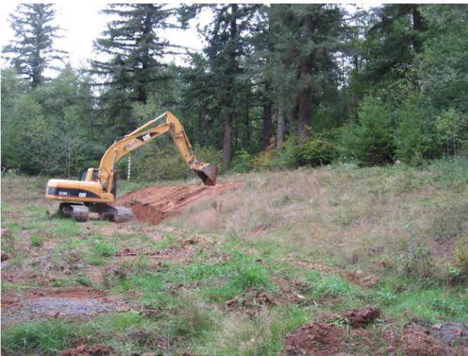
Excavating berm face
