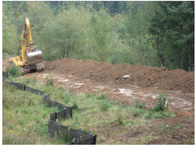
Excavating berm face
