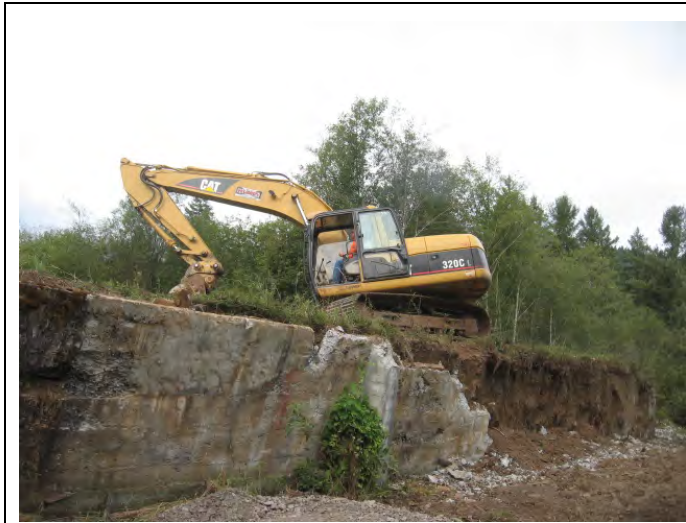
Dismantling and excavating berm along retaining wall
