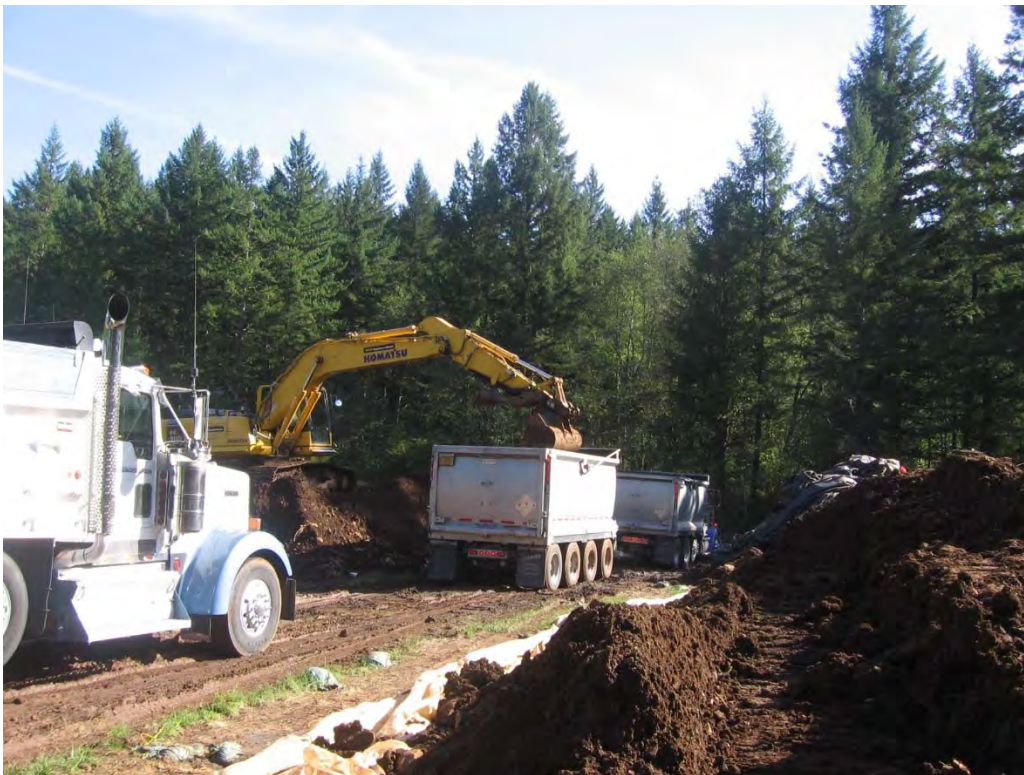
Loading Soil for Disposal, October 2010
