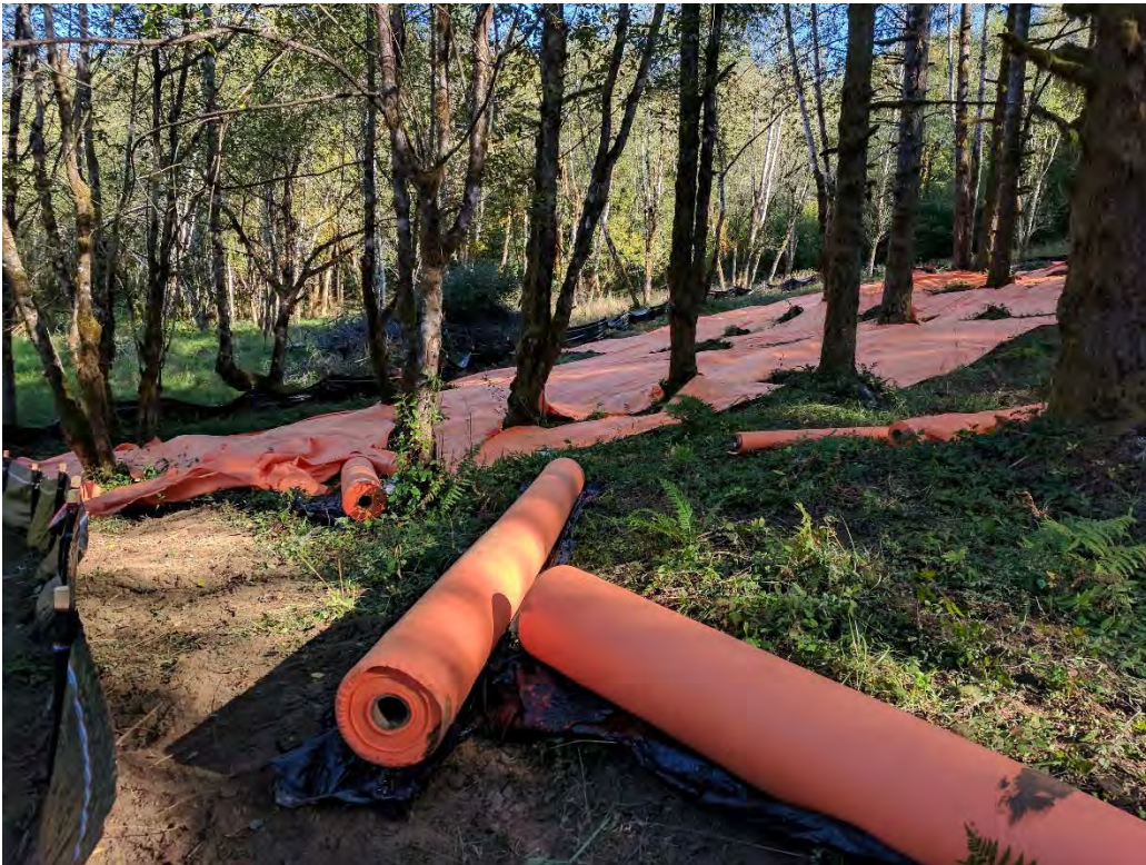
Installing demarcation geotextile, RAU 2A-16
