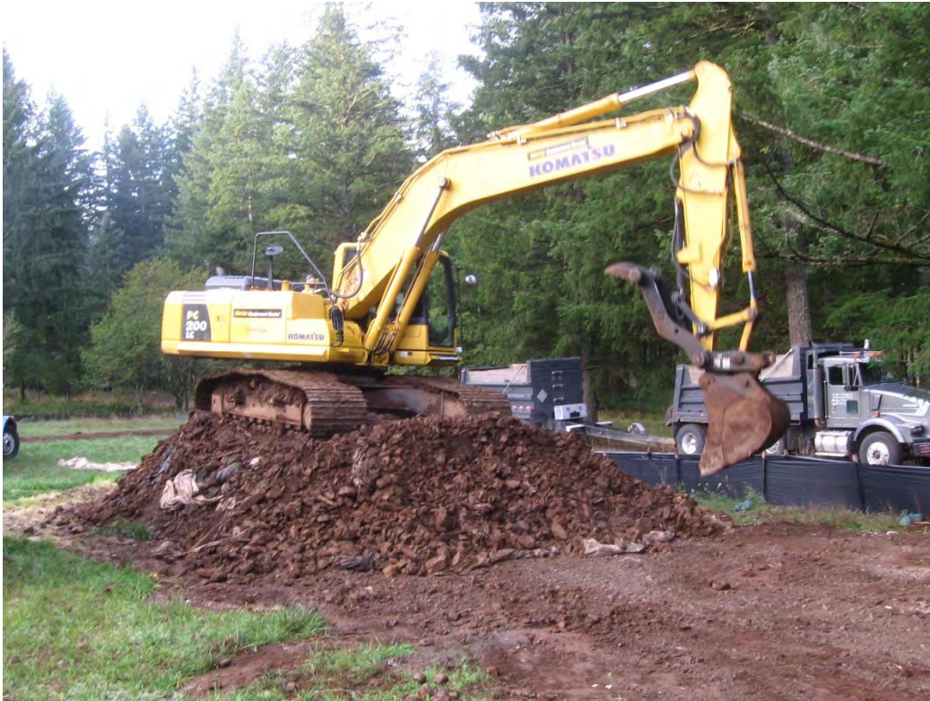
Loading Soil for Disposal, October 2010
