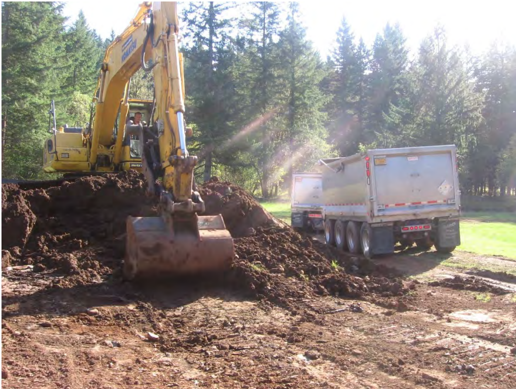
Loading Soil for Disposal, October 2010
