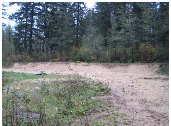
Erosion control mulching
