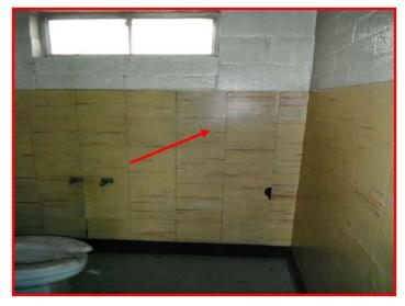
**Image 5:** Yellow 12-inch vinyl tile and associated black adhesive, located within the office restroom was identified through laboratory analysis to be an **ACM**
