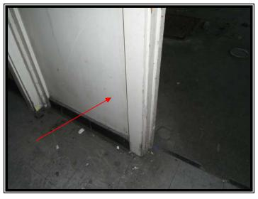
**Image 9:** Joint compound associated with gypsum wallboard was identified through laboratory analysis to contain less than 1% asbestos
