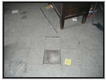
**Image 6:** Gray 9-inch vinyl tile and associated black adhesive, located within the office was identified through laboratory analysis to be an **ACM**
