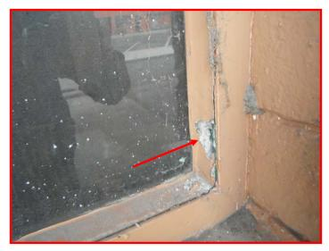
**Image 8:** Gray window putty was identified through laboratory analysis to be an **ACM**
