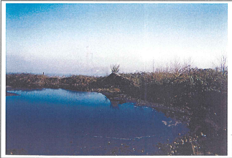
Photo 8. Settling pond with earthen berm facing east (2/12/04).
