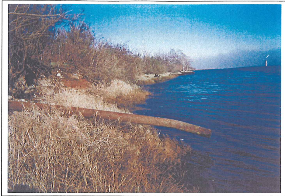
Photo 17. A 6-inch, steel, out fall pipe on the Sites shoreline (2/12/04).
