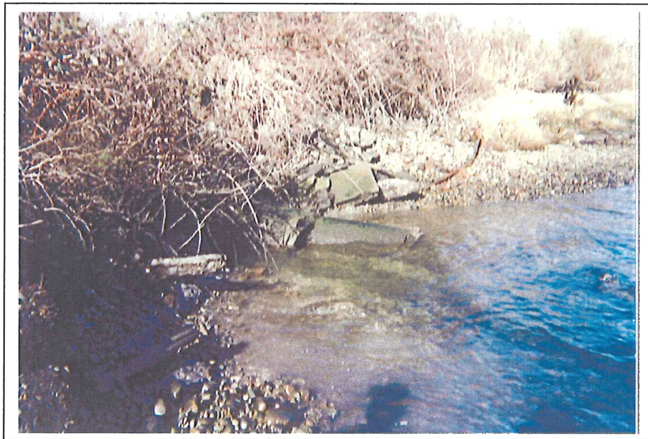
Photo 18. A 20-inch concrete out fall pipe on the Sites shoreline (2/12/04).
