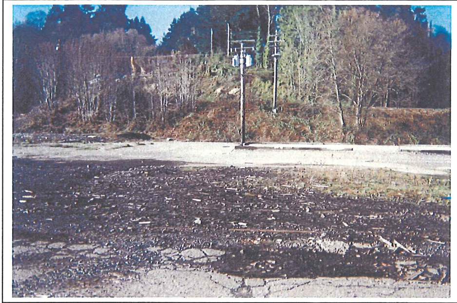
Photo 1. In the foreground, broken up asphalt with railroad. Center of photograph a concrete foundation protruding from former structure with electrical pole with transformer, facing west (2/12/04).
