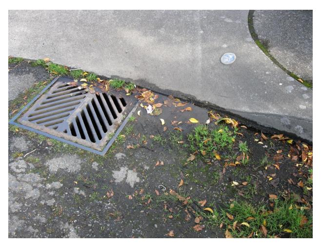
Note seep flow entering storm drain that discharges to surface water.
