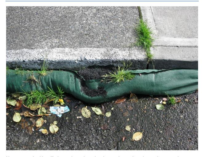
Note torn sock with spilled granular activated carbon and grass/weeds growing on sock.
