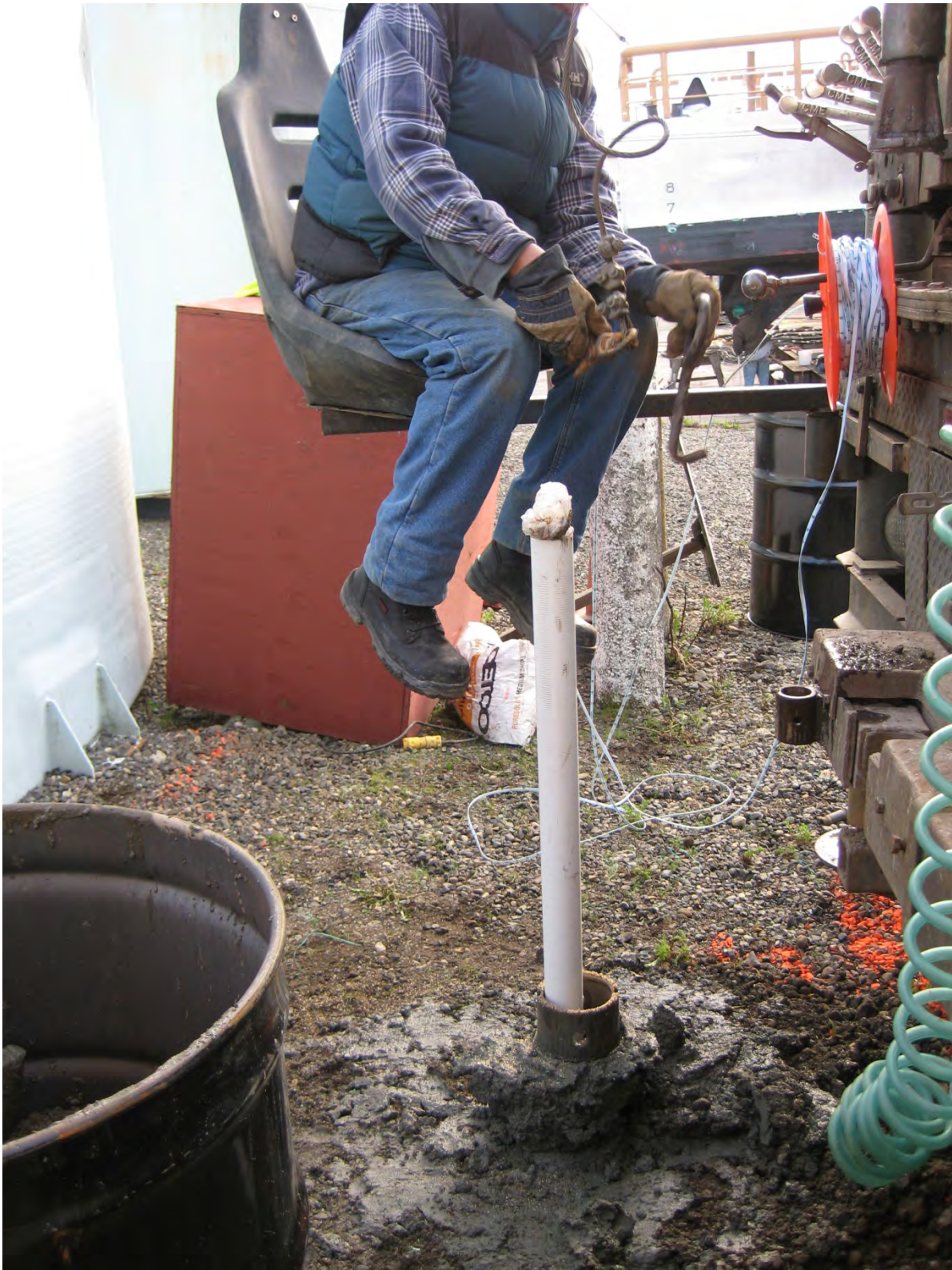
Photograph 7. Well installation at Monitoring Well MW-02A in the Northern Shoreline Area.
