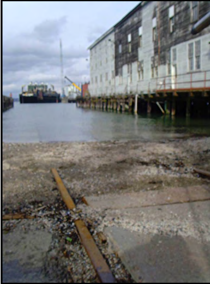
Figure 7. Marine rails (G) southwest of shops and loft (A).
