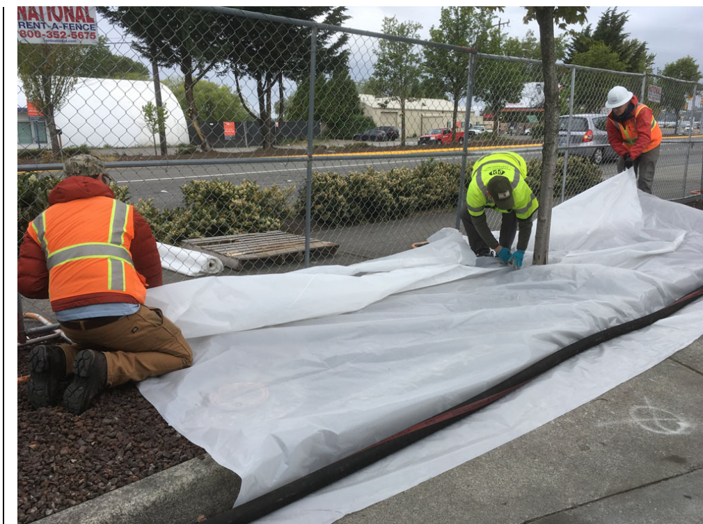
Photo #1: Setting up visqueen on gravel area adjacent to AS-1 prior to operation of the air sparge (AS) system.
