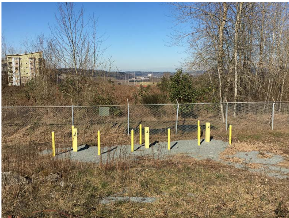
Photo 4: New gas probes near the property boundary.
