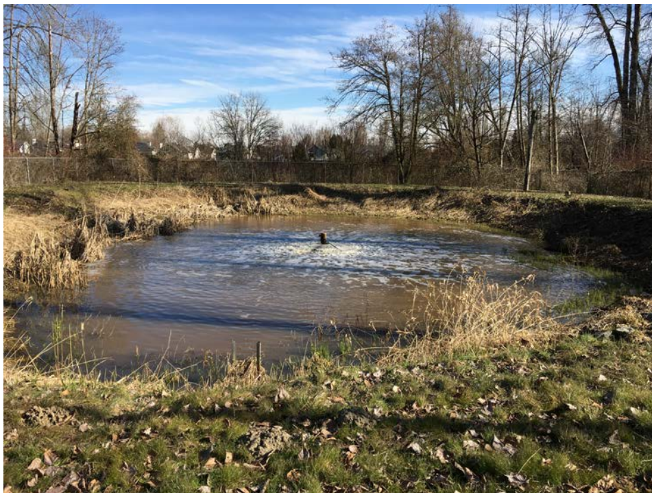
Photo 8: Lined leachate aeration pond that discharges to sanitary sewer.
