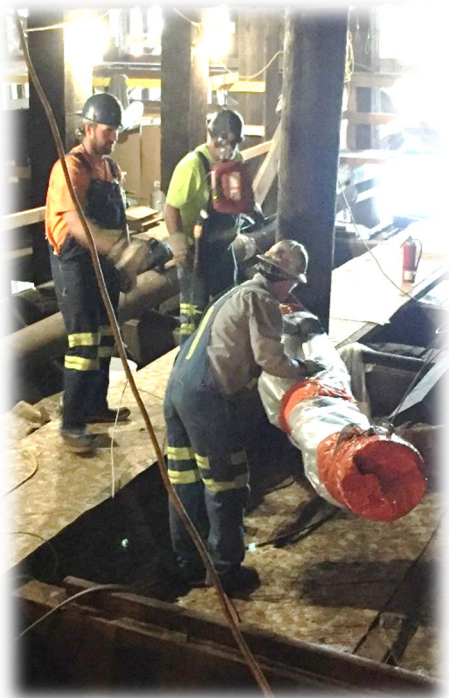
REMOVAL OF LINE 'E' END-SECTION
