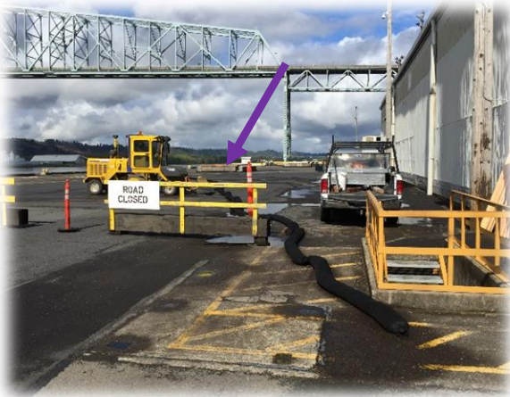
EAST (UPSTREAM) END OF PROJECT, AT STAIRWELL, SE CORNER OF TS2, LOOKING WEST. NOTE COMPOST WATTLE (TO DIVERT ANY EXCESS RUNOFF), SWEEPER, AND MAIN (CENTER) ACCESS HOLE IN BACKGROUND.
