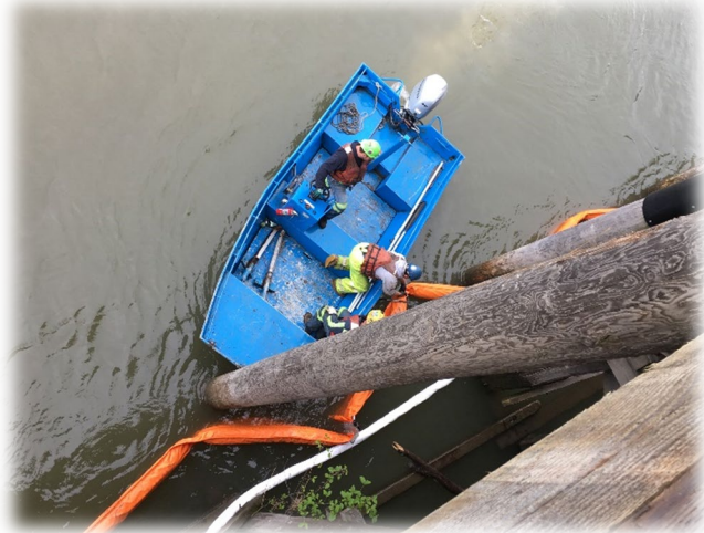
BOOM INSTALLATION
