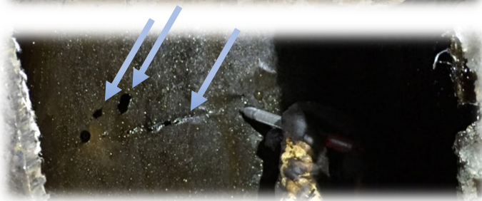
FIRST LEAK. LINE D, 75' WEST OF CENTER. NO SPILLS SECOND LEAK. LINE D, 60' WEST OF CENTER. NO SPILLS. NOTE PIPE PERFORATIONS AND CRACK.
