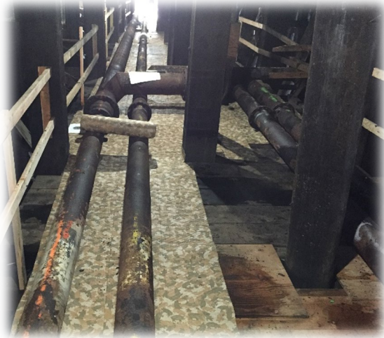
INSTALLATION OF NEW PIG 'HAMO' OIL-ONLY ABSORBENT MAT SURFACING UNDER DOCK.
