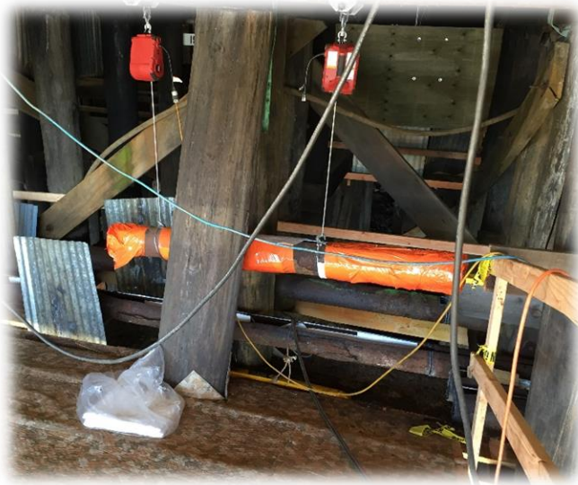
LIFTING PIPE NEAR BULLRAIL
