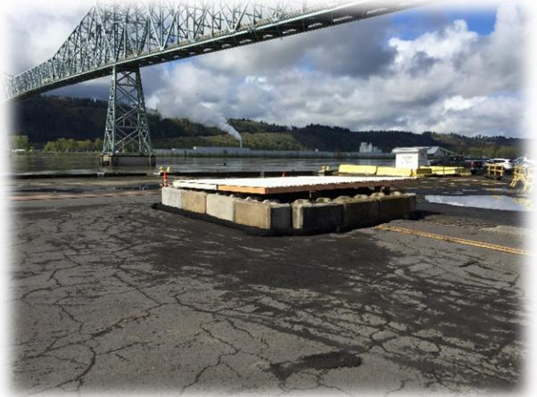
WEST ACCESS HOLE LOOKING S/SE. NOTE COMPOST WATTLE AND COVER. NOT SHOWN IS CLOSED-CELL BACKER-ROD UNDER BLOCKS.
