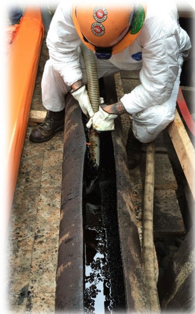
TROUGHED PIPE, W/ OIL. VACUUMING PIPE. SURFACE OPERATIONS.
