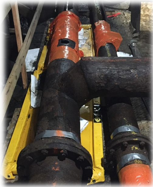
FIRST LEAK. LINE D, 75' WEST OF CENTER. NO SPILLS SECOND LEAK. LINE D, 60' WEST OF CENTER. NO SPILLS. NOTE PIPE PERFORATIONS AND CRACK.
