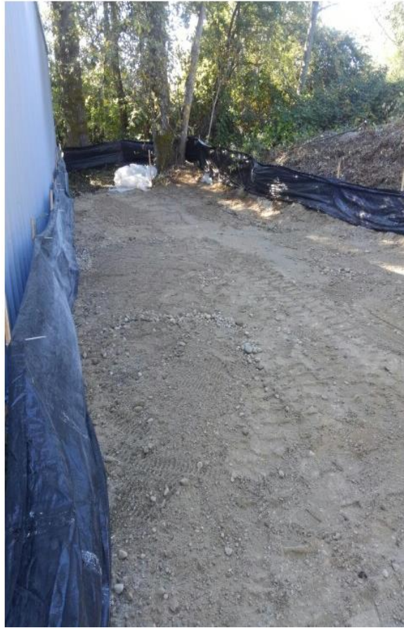
Backfill of side area
