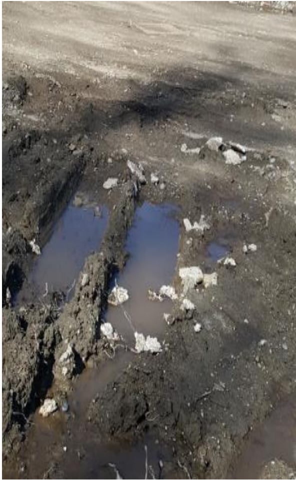
Soil displacement near SS-1
