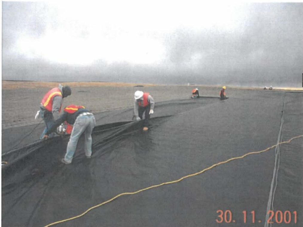
Field Lining Systems sewing geotextile.
