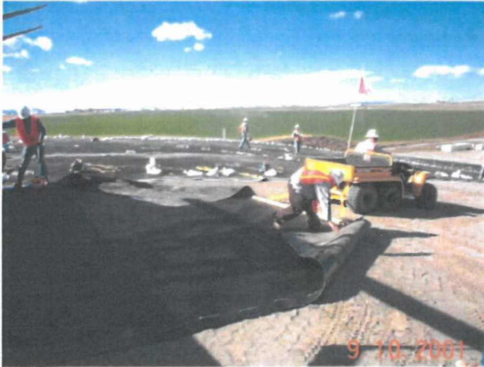
Deployment of 40 mil textured LLDPE geomembrane north slope MSW area.
