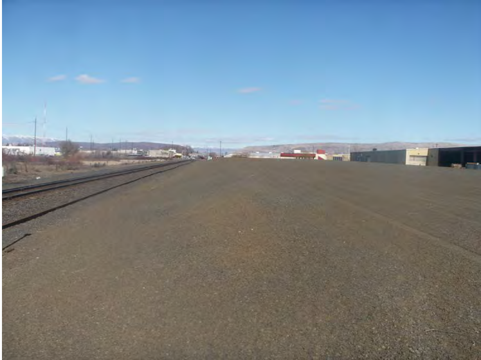
Photograph 7: Western side and top of BNSF main cell, looking north.
