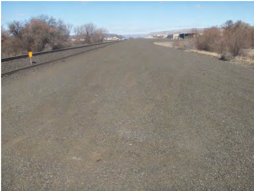
Photograph 2: Top of BNSF cell finger at southern end, looking north.
