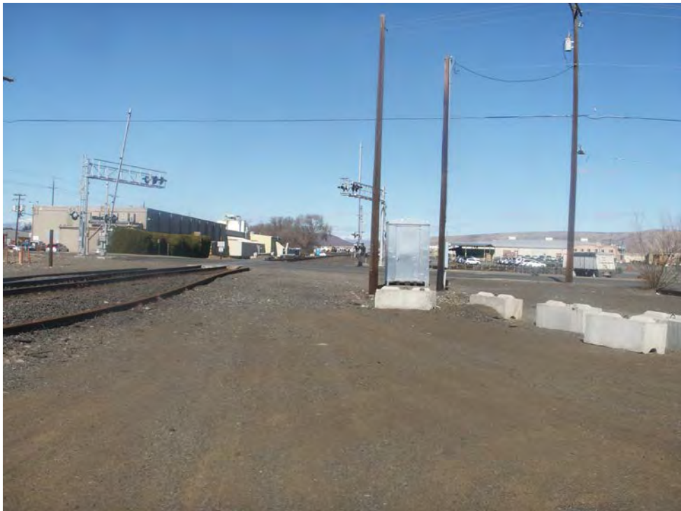
Photograph 18: Northern entrance to BNSF cell from East Washington Avenue, looking north.
