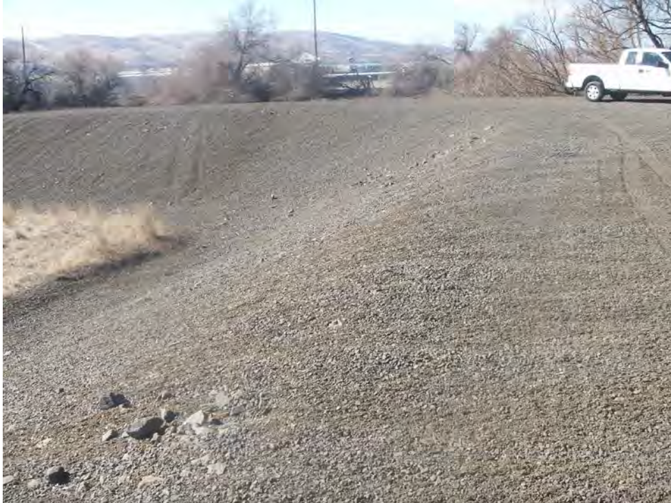
Photograph 9: Southeastern side of BNSF main cell and cell finger with Quad tracks, looking west.
