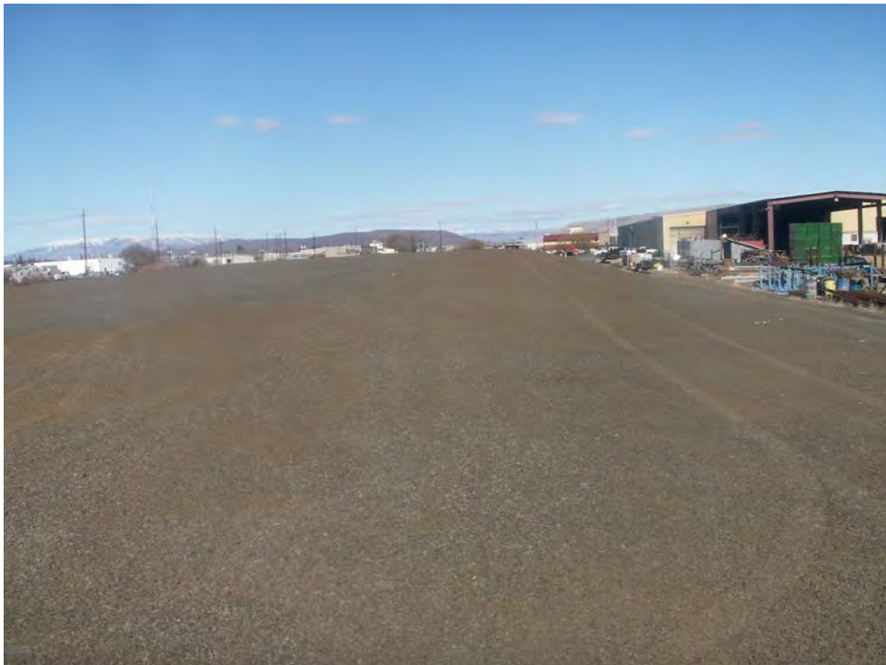
Photograph 10: Northeastern side of BNSF main cell, looking north.
