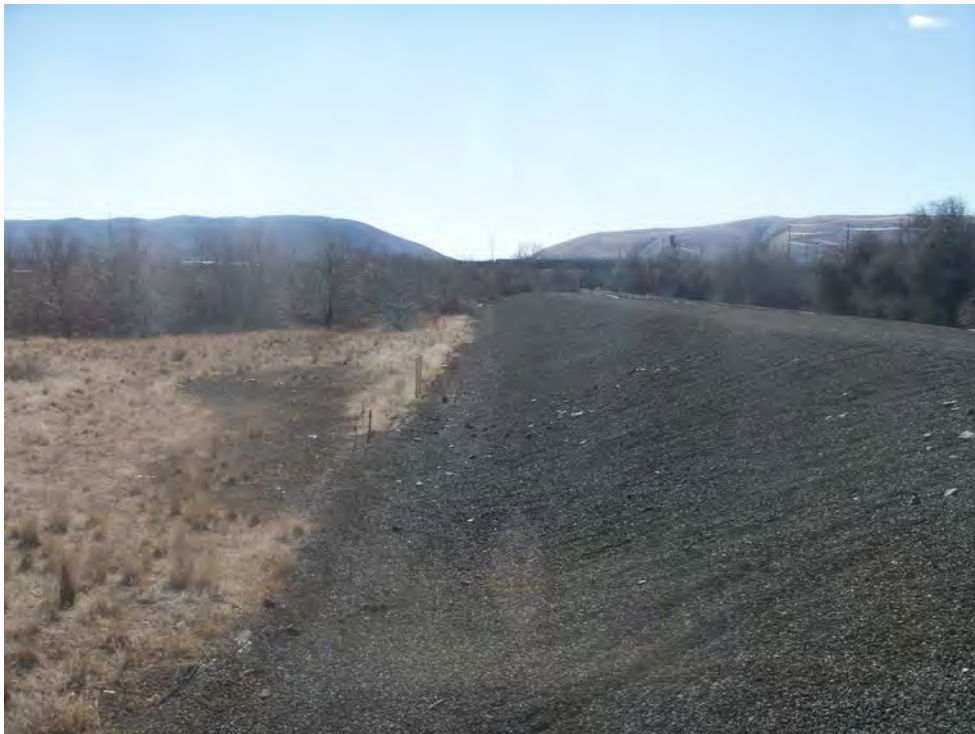
Photograph 6: Eastern side of BNSF cell finger and monitoring well MW-12, looking south.
