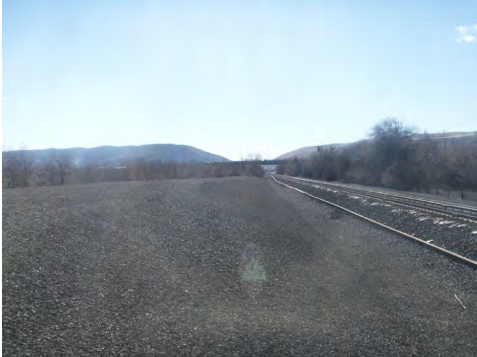
Photograph 5: Western side of BNSF cell finger and BNSF tracks, looking south.
