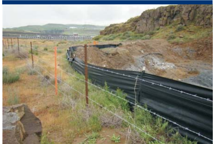
Photo 10 Landfill southern extent and US Army Corps border. Monitoring well MW-2 in top center of picture.
