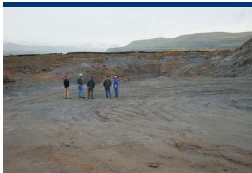
Photo 4 Site walk looking at silt fence border of US Army Corp property and extents of landfill.
