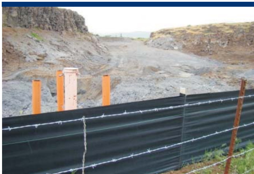
Photo 3 Basalt wall to south, entrance to landfill on opposite side, monitoring well MW-3 close up.
