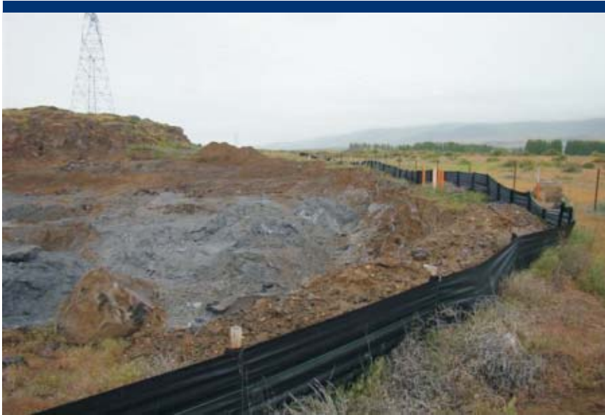
Photo 9 Landfill north boundary and silt fence along Army Corps property. Monitoring well MW-3 in right center of picture.
