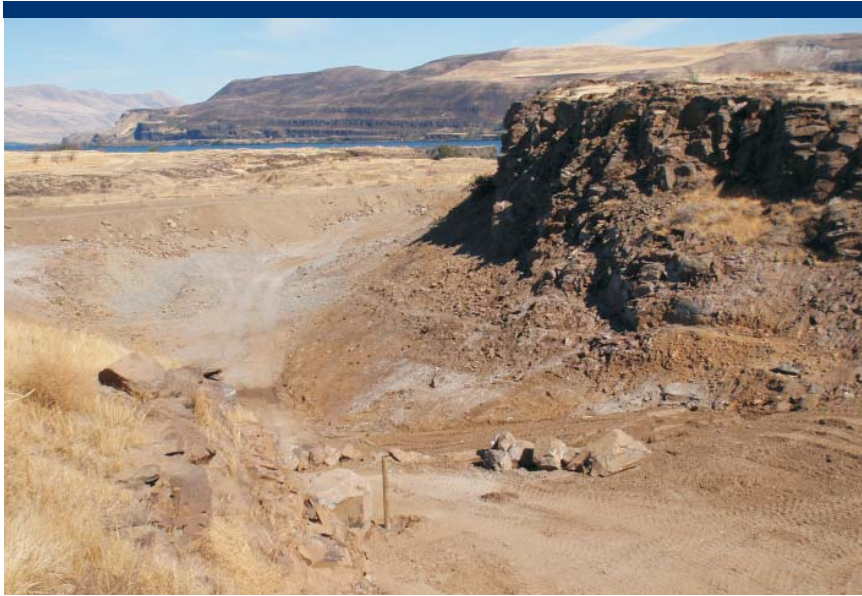
Photo 21 West entrance to the landfill post removal view. Note the fence post and large rocks to be used to gate the west entrance.
