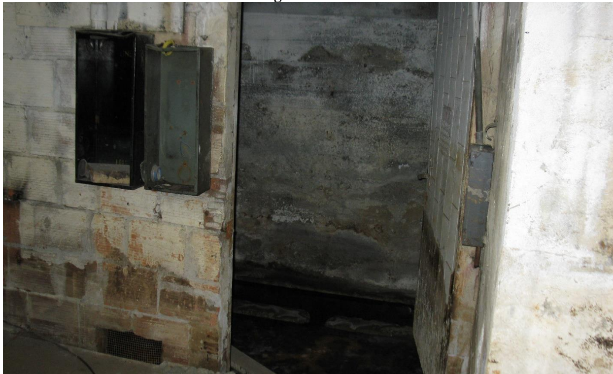
Photo 6: Site Building Basement/Former Underground Storage Tank Decommissioned Location and Concrete Flooring on the Contaminated Soil
