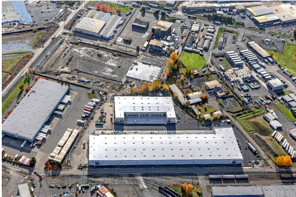
Photograph 5. Aerial of property; view to the southwest. Building A is in the lower portion of the photo, and Building B is adjacent to and southwest of Building A.
