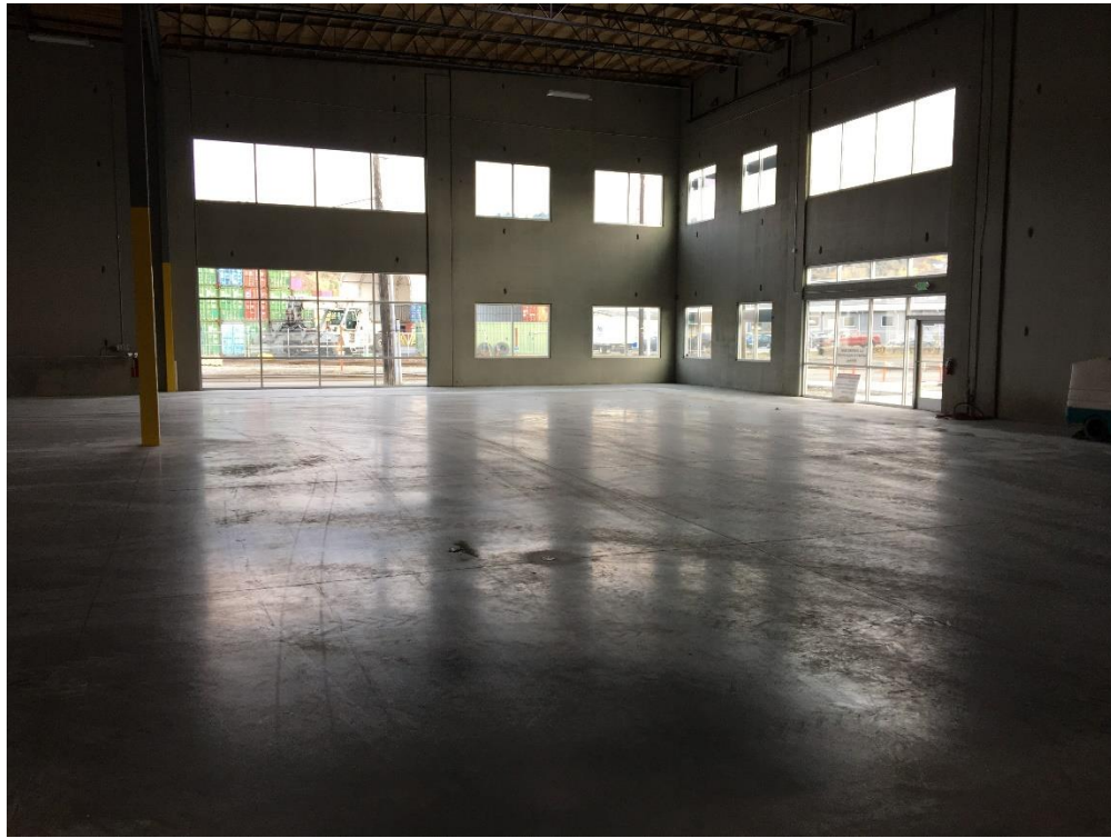
Photograph 7. Building A interior; northeast office node.
