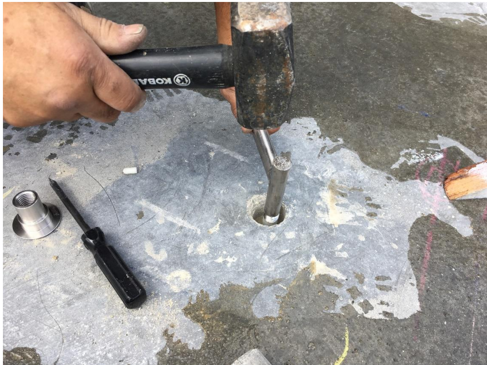
Photograph 2. Hammering vapor pin in place.
