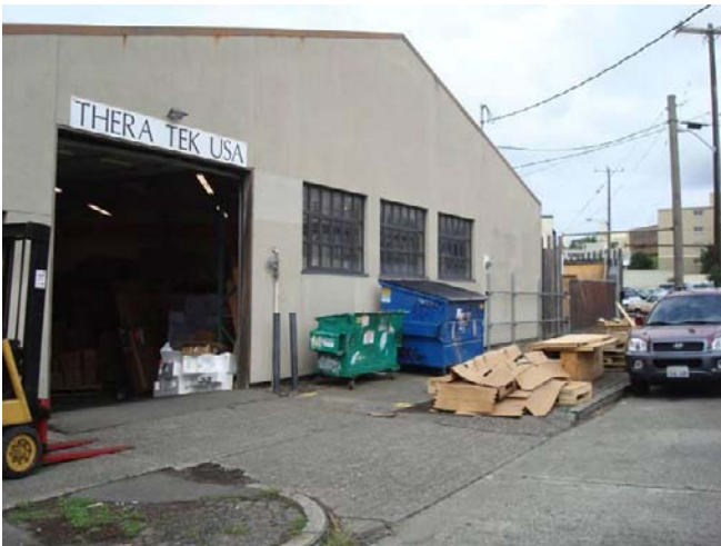
Photograph 11. Looking northwest at the building located on the north-adjointing property.
