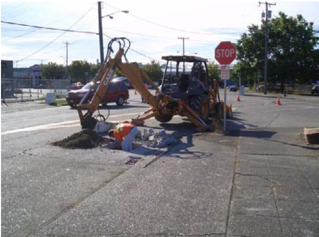
Photograph 9. Looking southeast at magnetic anomaly investigation.
