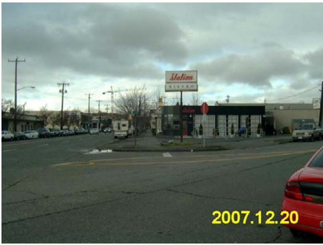
Photograph 1. Looking northwest at the Property from the southeast.
