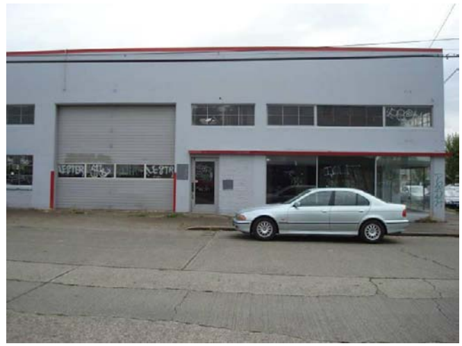
Photograph 8. Looking east across 17 th Avenue Northwest to the vacant former service garage.
