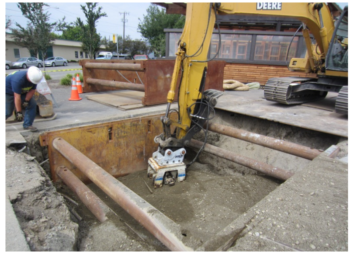
Photograph 8. Hydraulic tamping of backfilled portion of excavation.
