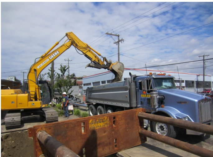
Photograph 5. Direct loading of soil for off-site removal.
