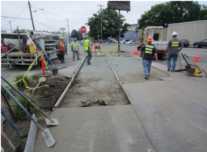
Photograph 9. Backfilled excavation extent.
