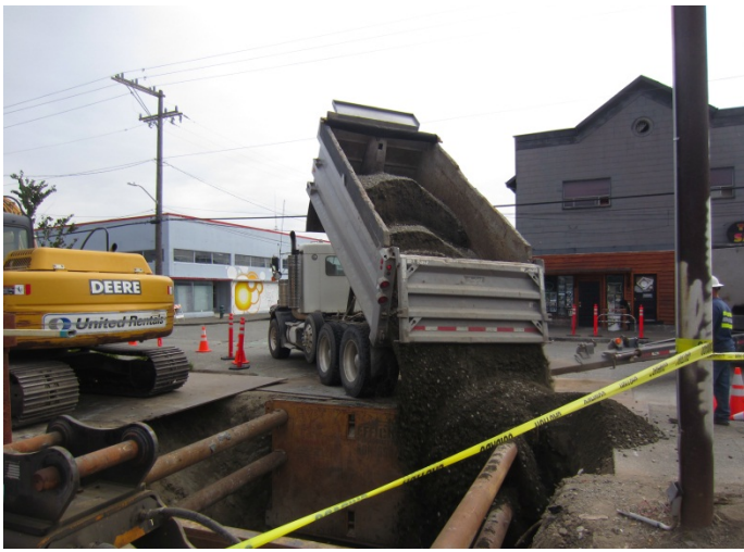
Photograph 7. Clean fill imported to Site.
