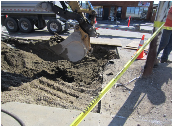
Photograph 1. Removing clean overburden.
