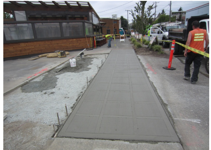
Photograph 10. Restoring sidewalk and parking lot surfaces.
