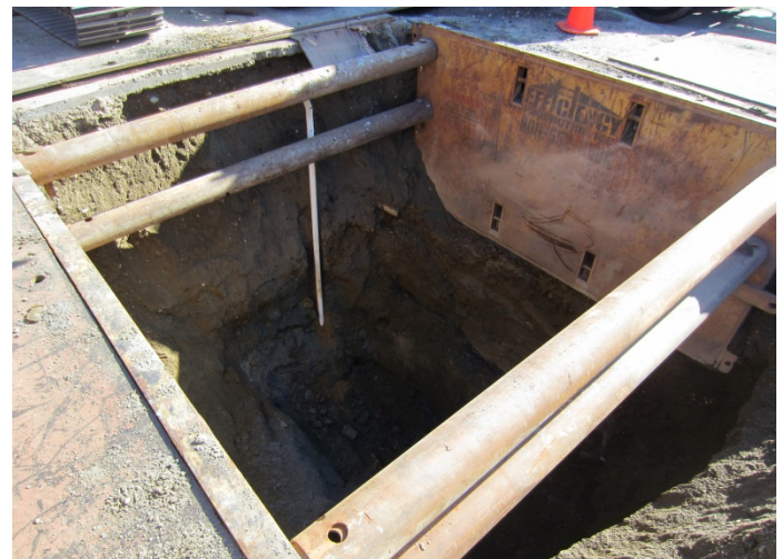
Photograph 6. Excavation of an approximate 100-square-foot "cell."
