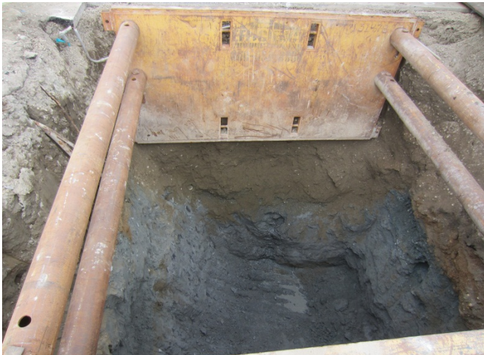
Photograph 3. Trench-box installed as an added safety measure.
