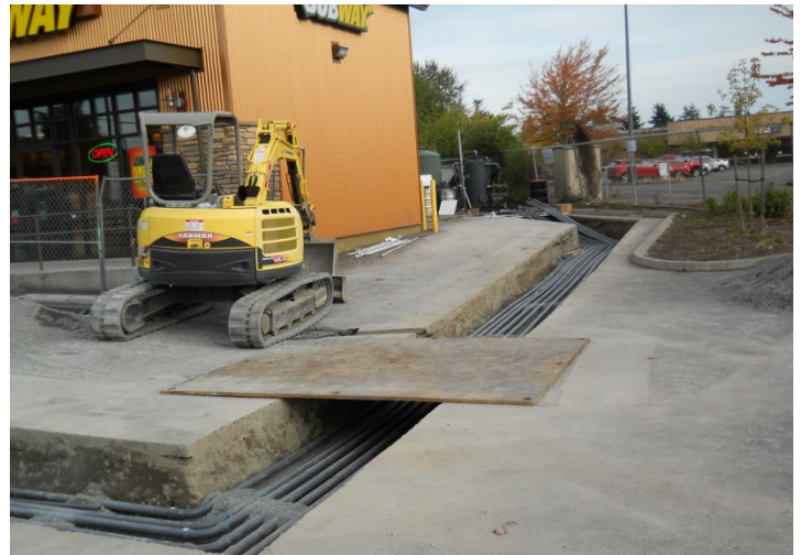
Photograph 16. Water and SVE lines in main trench.
