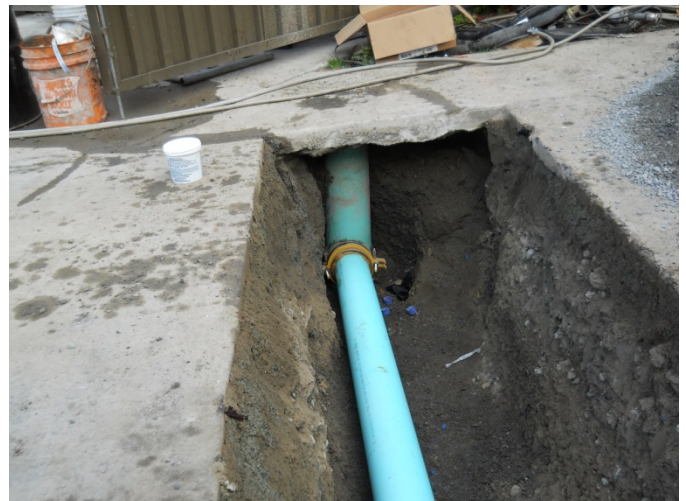
Photograph 18. Sewer connection.
