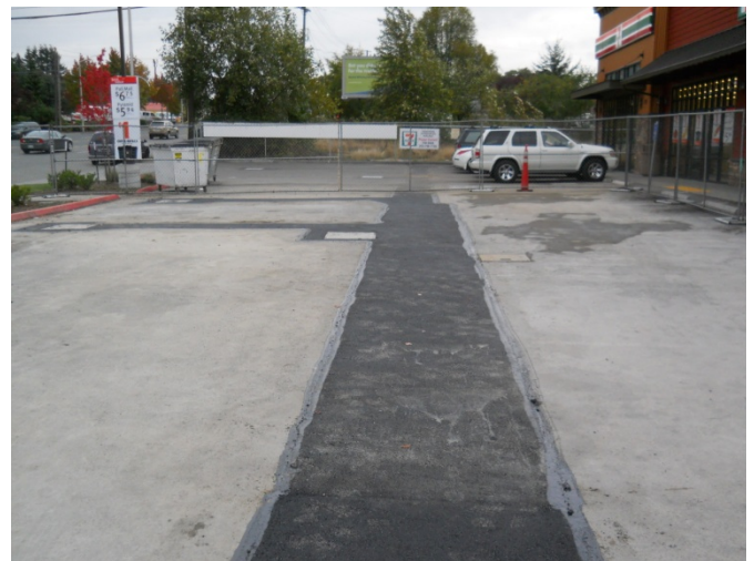
Photograph 22. Asphalt restoration for southern half of parking lot.
