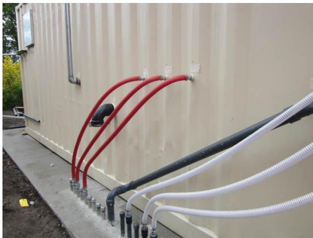
Photograph 27. Connections from sub grade to above ground piping for air, water, and sewer.
