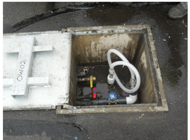
Photograph 26. Connections from sub grade to above ground piping for SVE.
