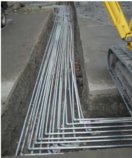
Photograph 15. Air delivery lines and electrical signal lines in south side of the parking lot (view looking north).
