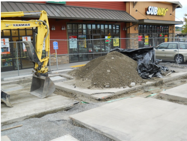
Photograph 11. Placement and compaction of back fill with warning tape exposed.
