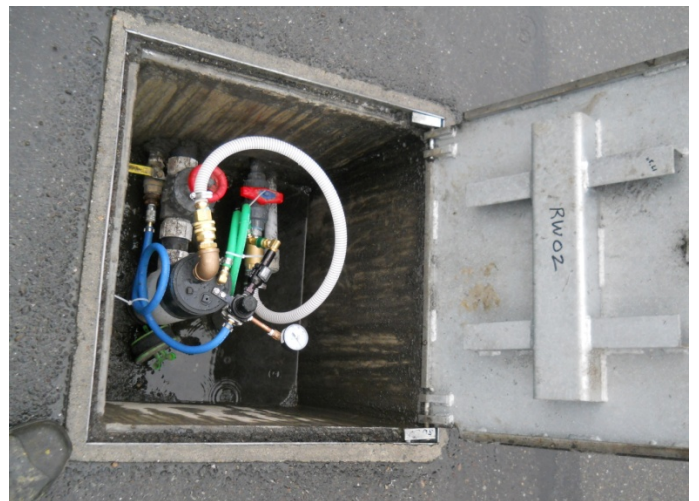
Photograph 34. Completed wellhead for RW02.
