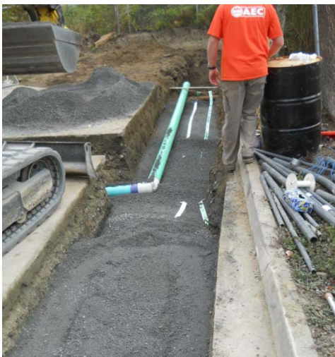
Photograph 21. Sewer tie in location, backfill, and warning tape.
