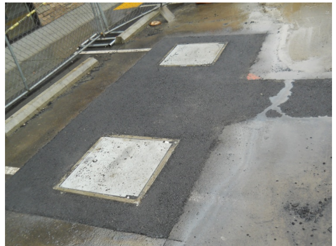
Photograph 12. MW08 and RW08 asphalt restoration.
