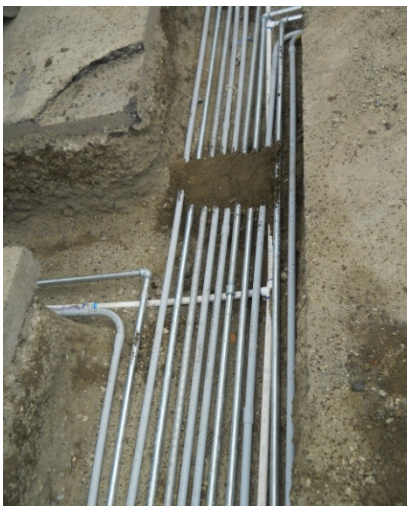
Photograph 9. Air delivery lines and electrical conduit in main trench at RW04 branch.
