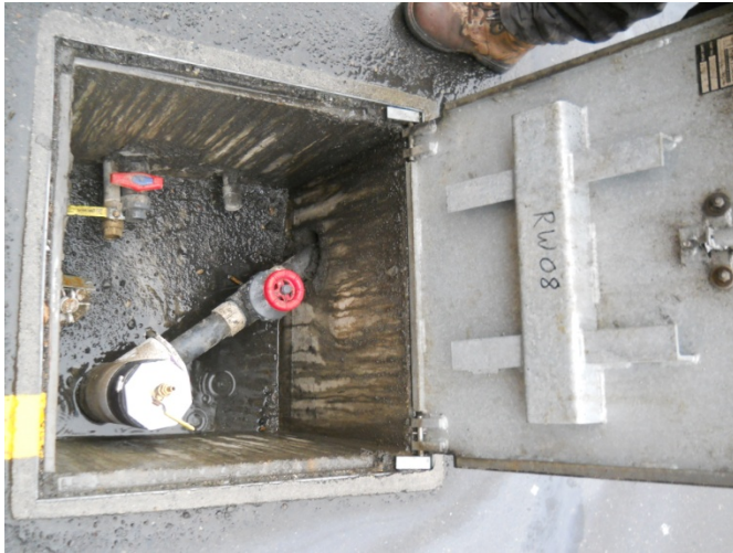
Photograph 31. Completed wellhead for RW08.
