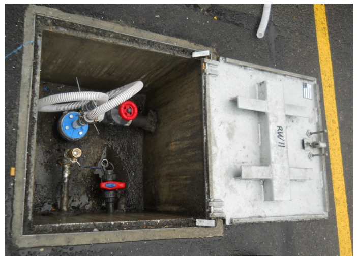
Photograph 30. Completed wellhead for RW11.
