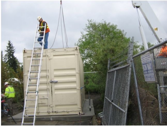
Photograph 25. Placement of the connex box.
