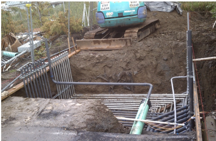
Photograph 23. Piping layout under remediation system concrete pad.
