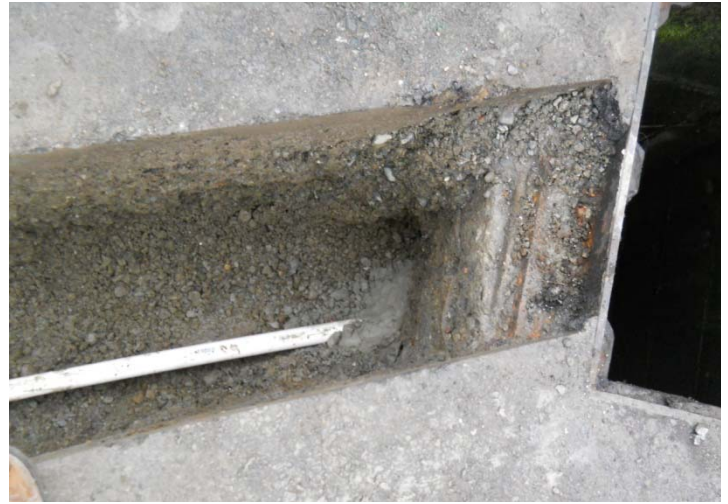
Photograph 14. Drain line penetration into storm drain.
