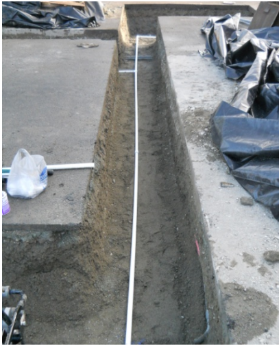
Photograph 7. Showing vault drain line from RW01 to RW03.
