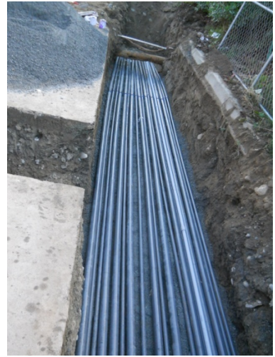
Photograph 20. SVE, water, and electrical feed.
