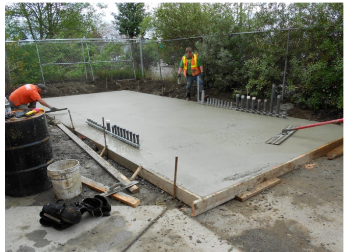
Photograph 24. Remediation system compound pad.
