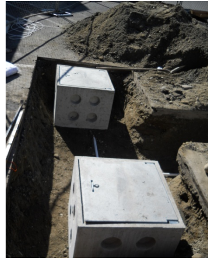
Photograph 8. MW08 and RW08 vaults and drain line.
