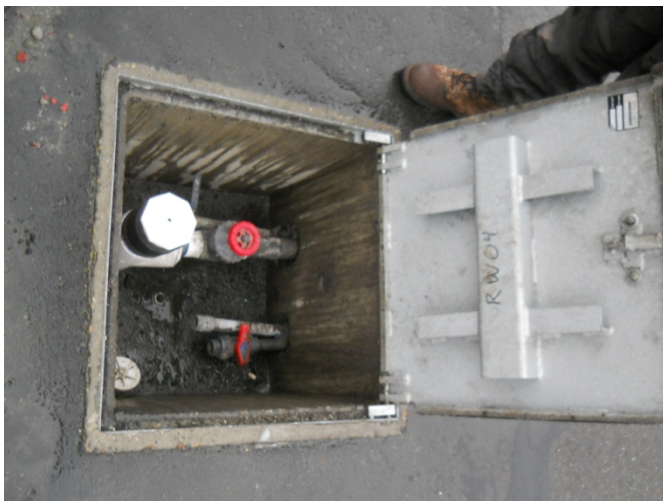
Photograph 33. Completed wellhead for RW04.
