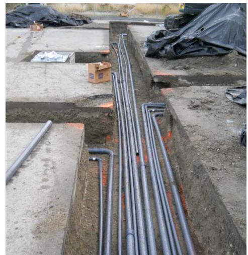
Photograph 10. SVE and water lines in main trench at RW04 branch (view looking north).
