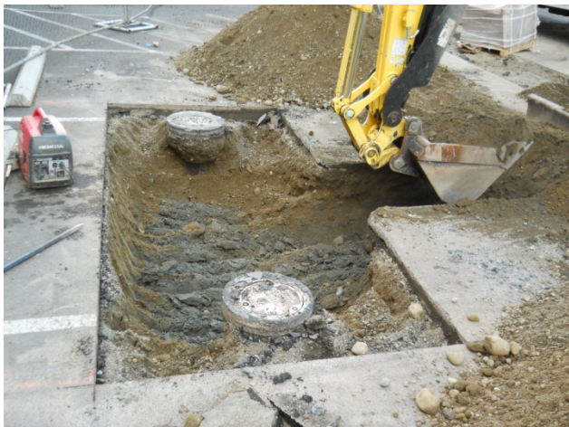
Photograph 5. Trenching near MW08 and RW08.
