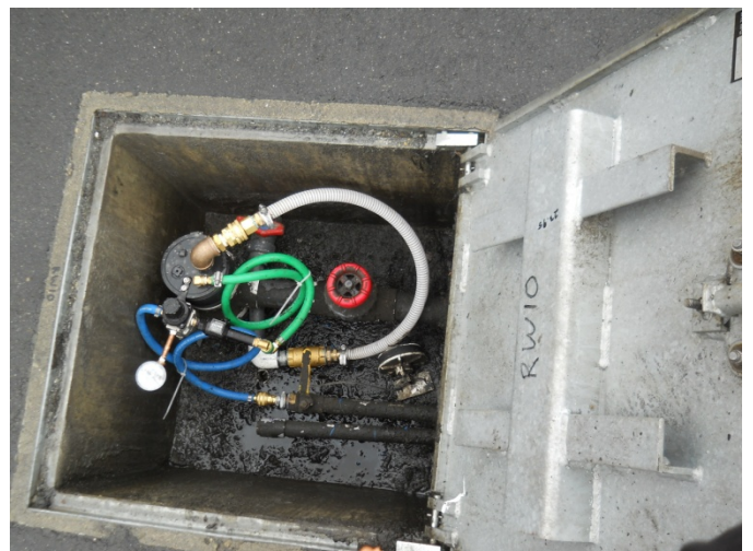
Photograph 36. Completed wellhead for RW10.
