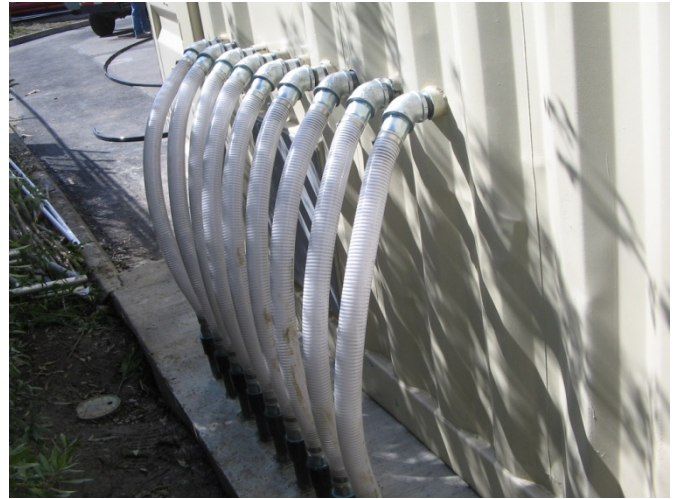
Photograph 26. Connections from sub grade to above ground piping for SVE.
