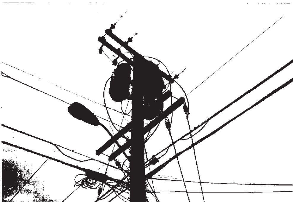
Photograph 4. A view of three pole-mounted transformers.
