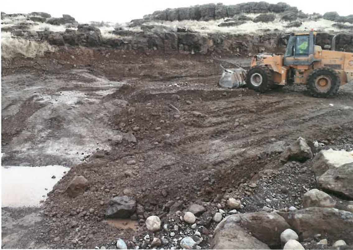
Photo 2. Soils scraped to bedrock (left) and excavator performing that process.
