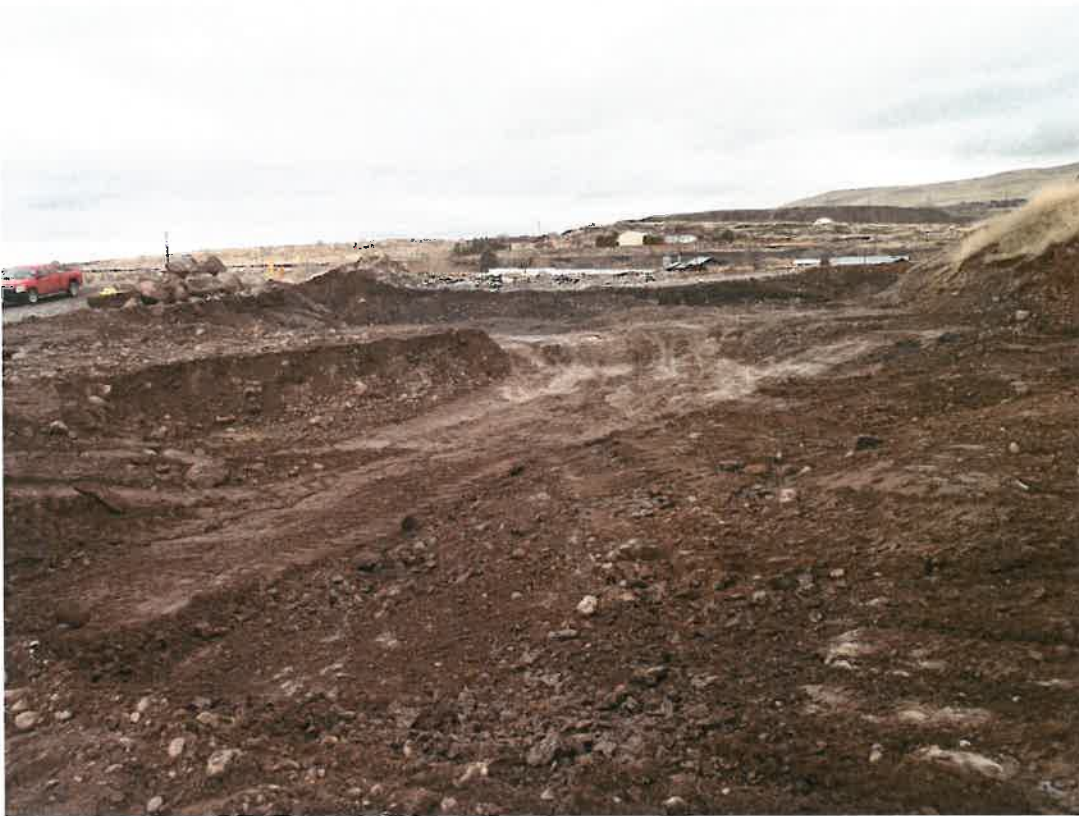
Photo 1. Rough excavation, elevated arsenic soil removal, Ephrata Landfill.
