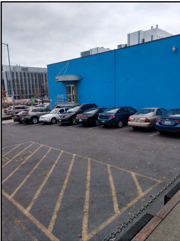
Photograph 2 – North Exterior and Entrance, looking southeast.
