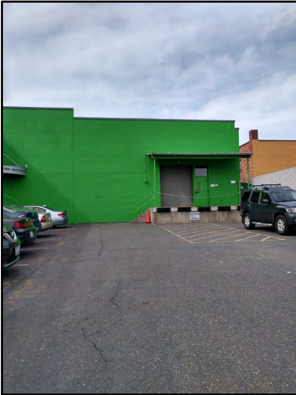
Photograph 1 – East Exterior and Loading Dock Area, looking west.
