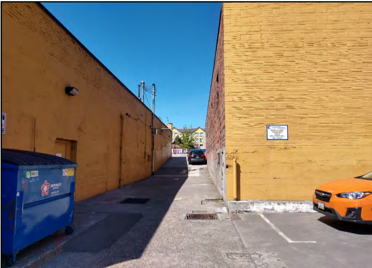
Photograph 14 – North Exterior and Alley – looking west.
