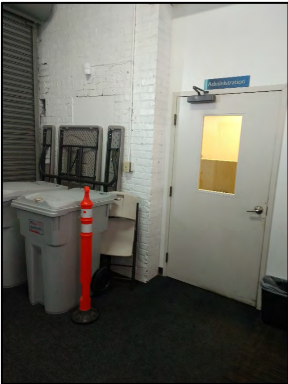
Photograph 12 – Interior Loading Dock Area, looking southeast.
