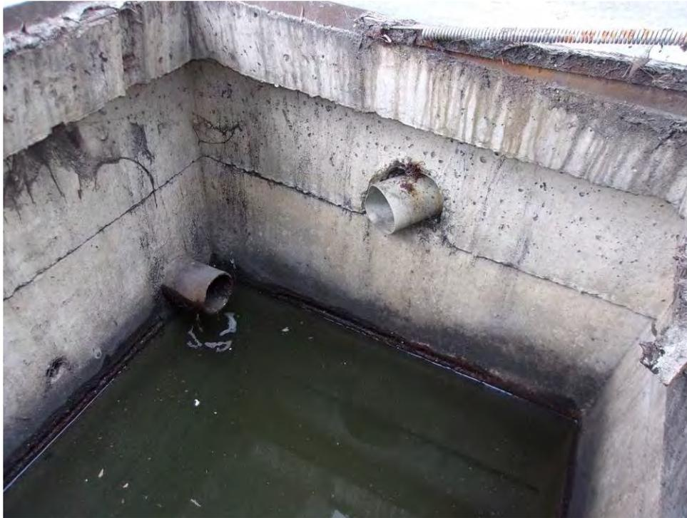
Photo 13: Sand separator (concrete vault) that collects parking garage stormwater in the northeast corner of the site.
