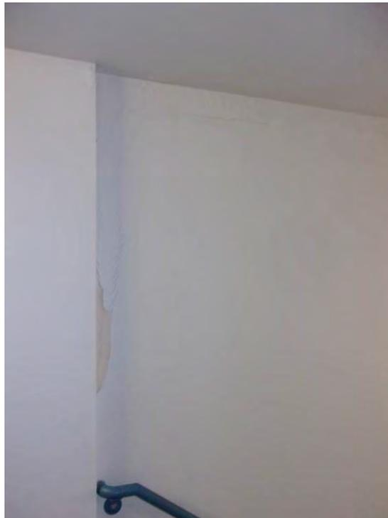
Photo 12: Peeling paint and light brown staining observed in stairwell #2.
