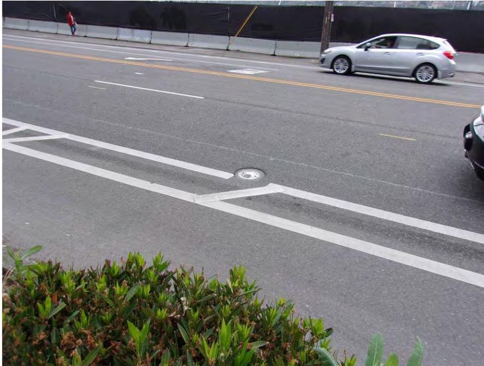
Photo 19: Monitoring well installed in the west side of Dexter Avenue North (adjacent to the northeast side of the site).
