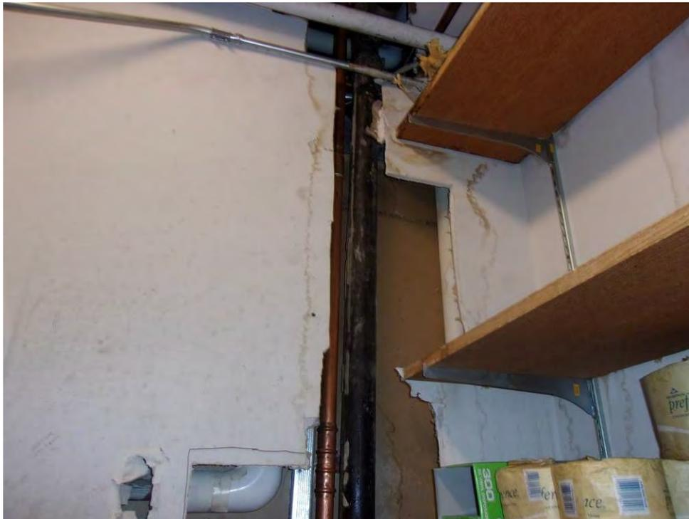
Photo 18: Light brown drywall staining in janitorial closet.
