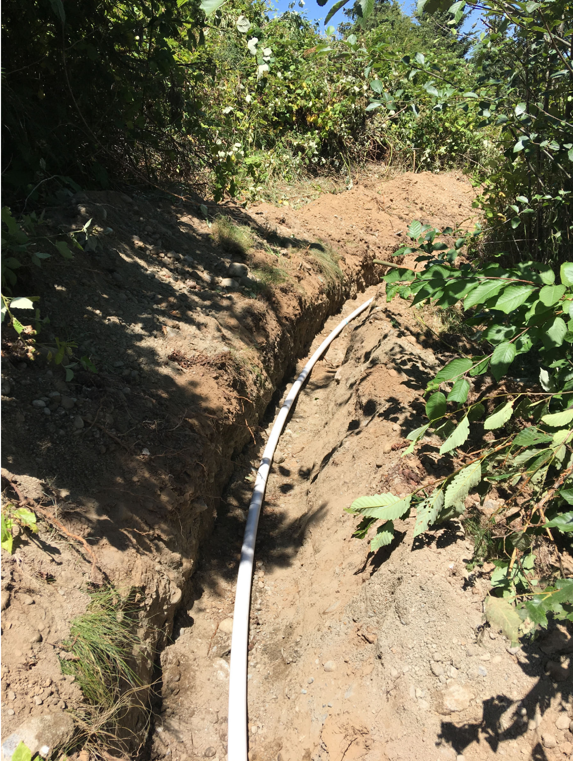
PVC Discharge Pipe to Leachate Manhole
