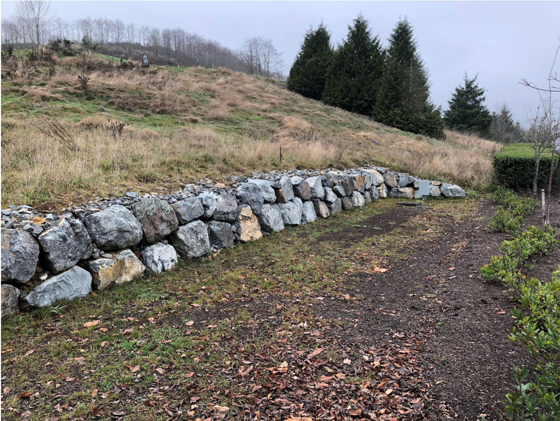
Completed Interception Trench (Dec. 5, 2019)
