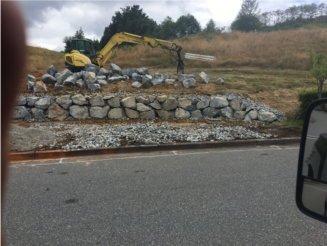
Construction of Rock Wall
