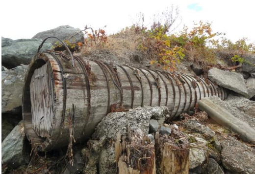
Pipe C (Outfall 002) at shoreline
