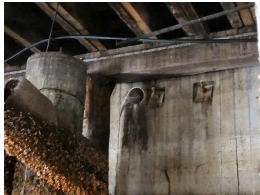
Pipe L (8-inch PVC)
