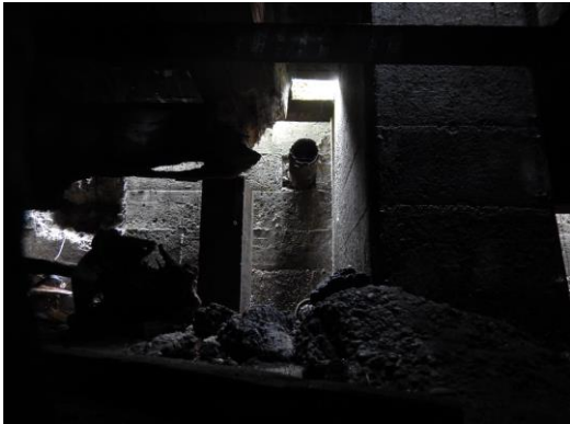
Pipe D (4-inch steel)
