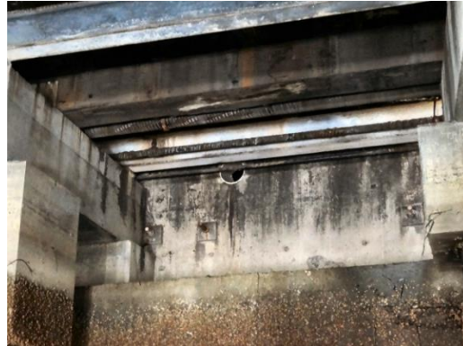
Pipe H (8-inch steel)
