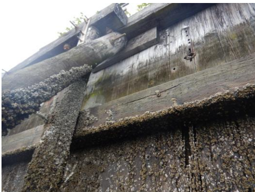
Pipe N (4-inch steel)
