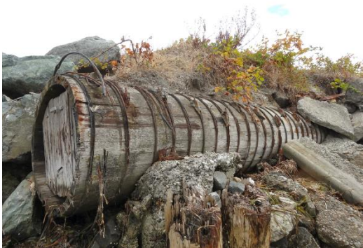
Pipe C (Outfall 002) at shoreline
