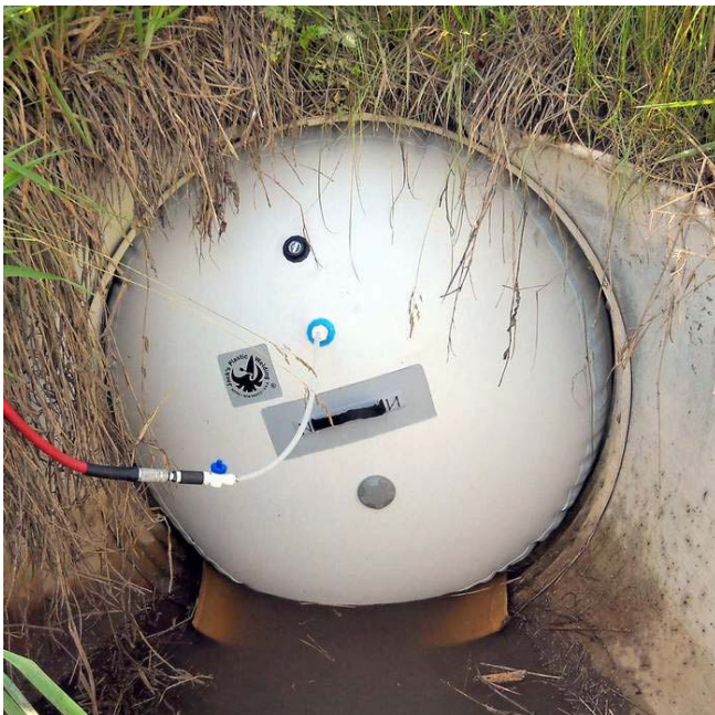
Photograph 2. Pneumatic Pipe Plug Application
