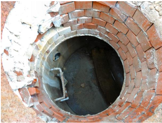
Lateral Pipe Entering City CSO Line at Easternmost Manhole on K-C Property
