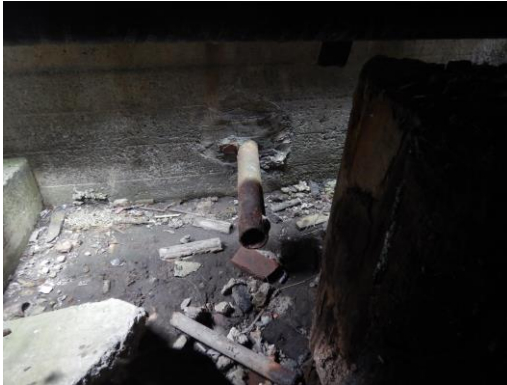
Pipe G (4-inch steel)
