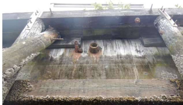
Pipes P (6-inch steel) and Q (2-inch steel)
