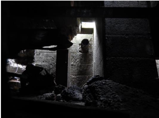
Pipe D (4-inch steel)
