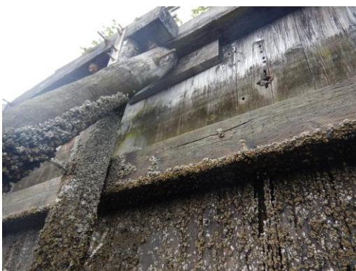
Pipe N (4-inch steel)
