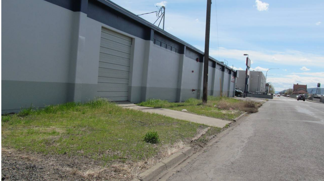
Photo 3: West Side of Building - from the northwest
