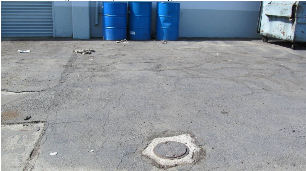
Photo 4: Monitoring Well (MW-2) East of Building – from the east
