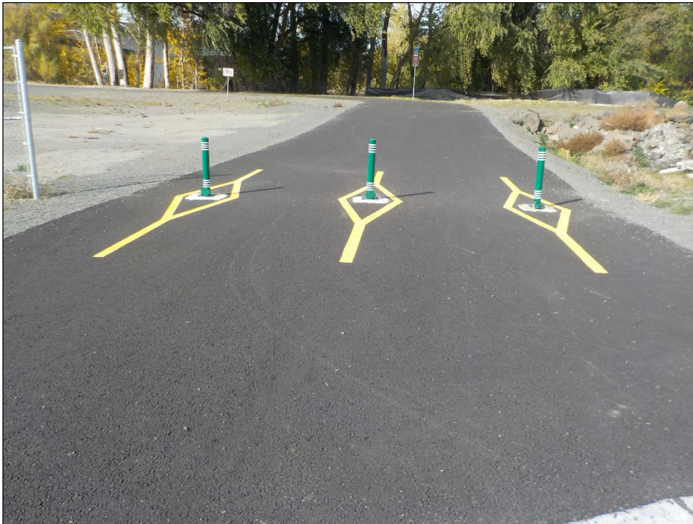
6. View of new section of Ben Burr Trail near northeast site boundary (looking northwest, toward Spokane River).
