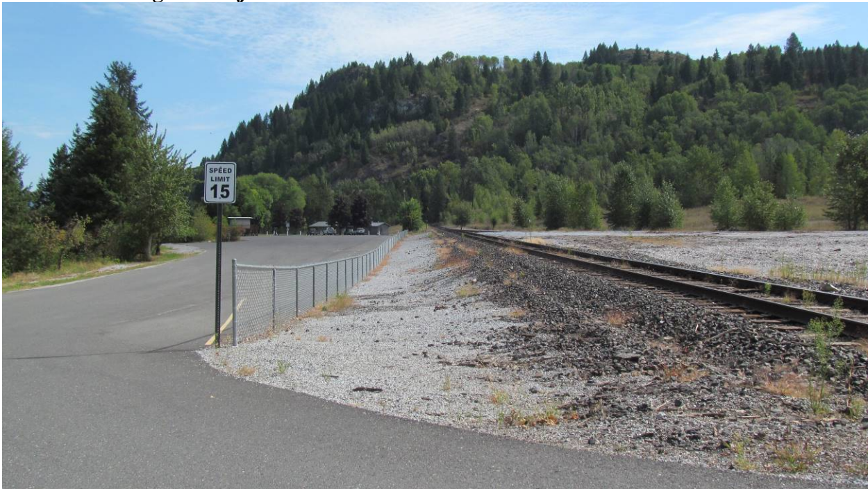
Photo 2: Fencing and Adjacent Railroad Tracks – from the southwest
