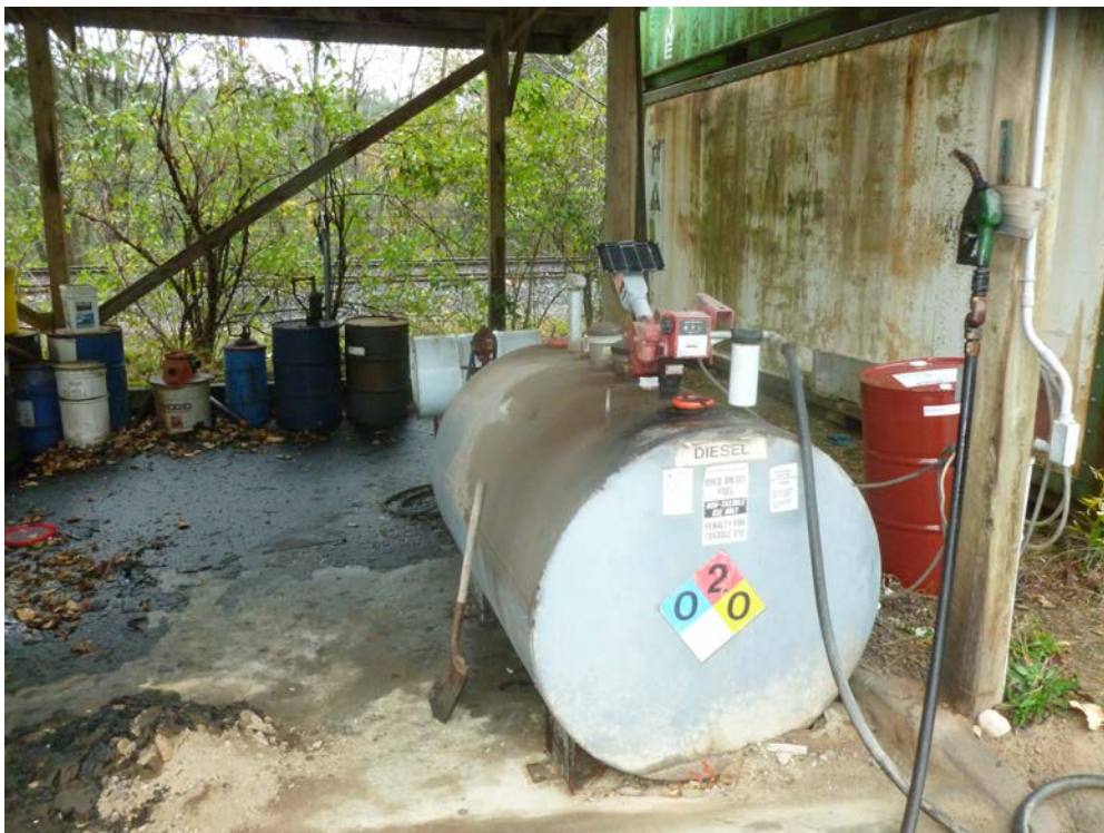
Photograph 4: Diesel AST and hazardous materials storage in equipment storage area.
