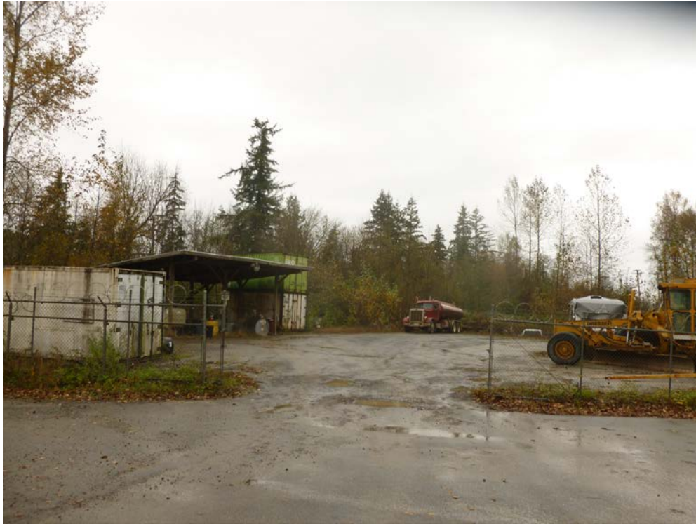
Photograph 3: Equipment storage area, aboveground storage tank (AST) and drums, looking east.
