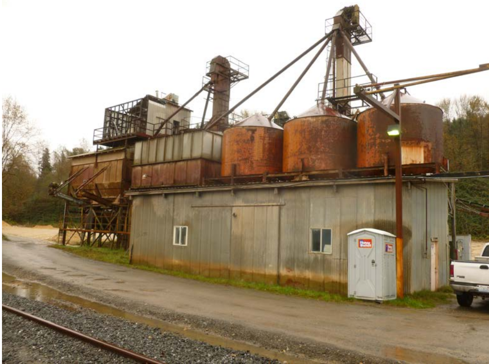
Photograph 1: Office building and former sand mining equipment, looking southeast.
