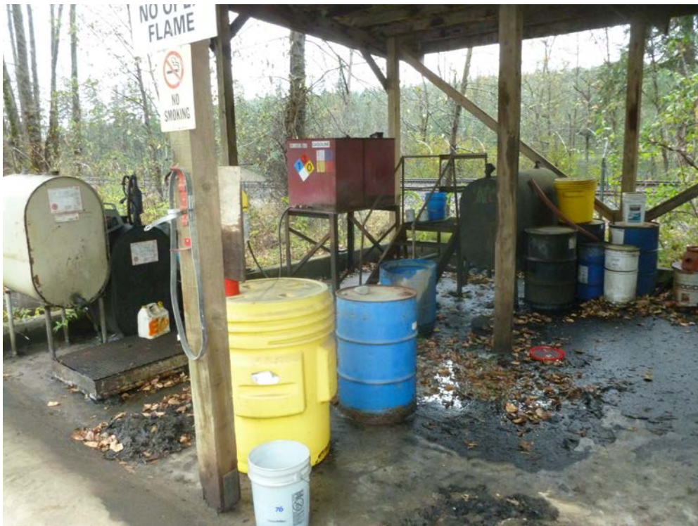
Photograph 6: Empty gasoline AST and other hazardous material containers under canopy in equipment storage area.
