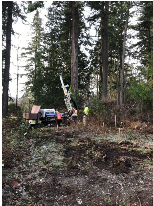
Photo 1 - Advancement of boring GB-14, an angle boring, completed along the western Property boundary.
