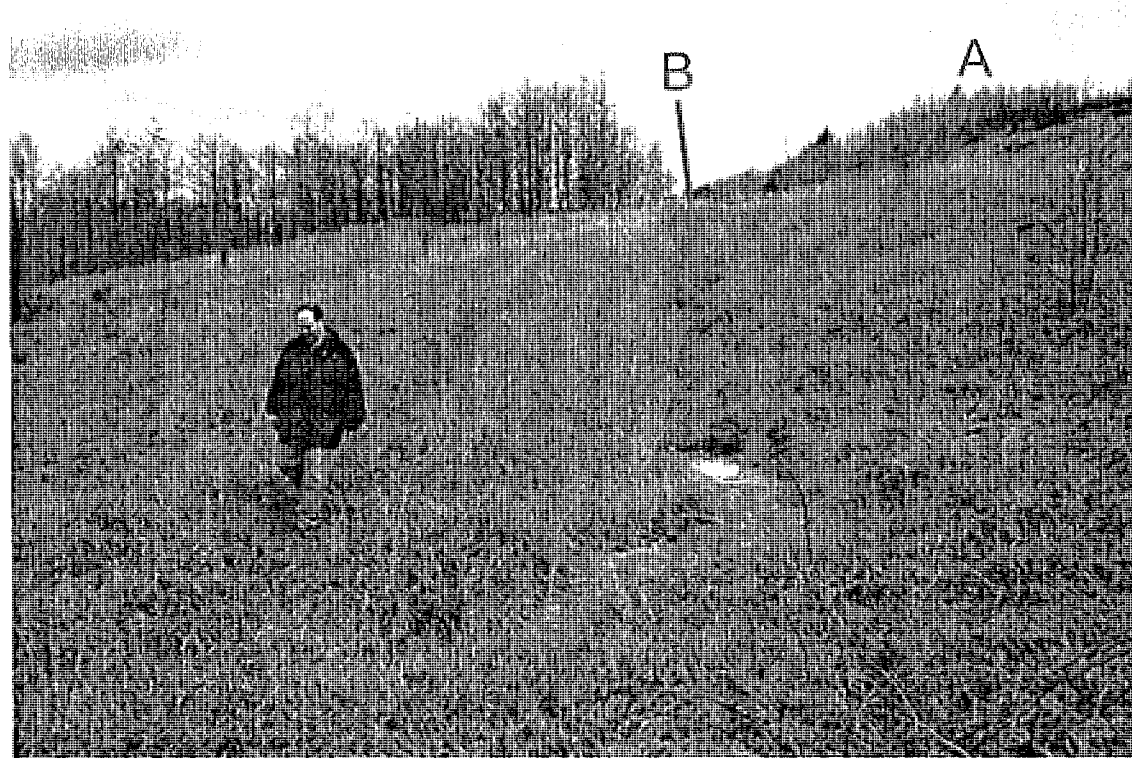
Photo 6-5 LDA. View to northeast from southwest part of LDA. Showing incised surface drainage patterns ("A-B") on LDA cap. Note exposed CKD in bottom of drainage at "A".
