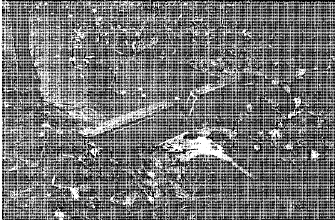
Photo 3-2 At Seepage Area. West side of LHR, below LDA. View to southwest of seepage water ponded behind flow monitoring weir.
