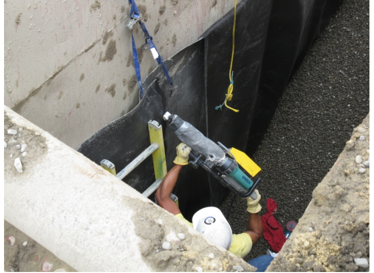
Extrusion welding of 8' x12' panel.
