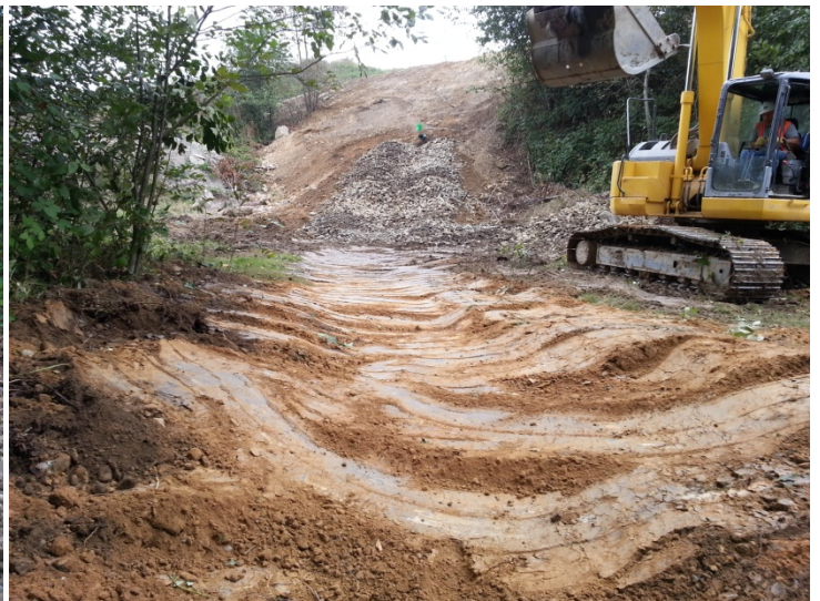
Bioswale excavation.
