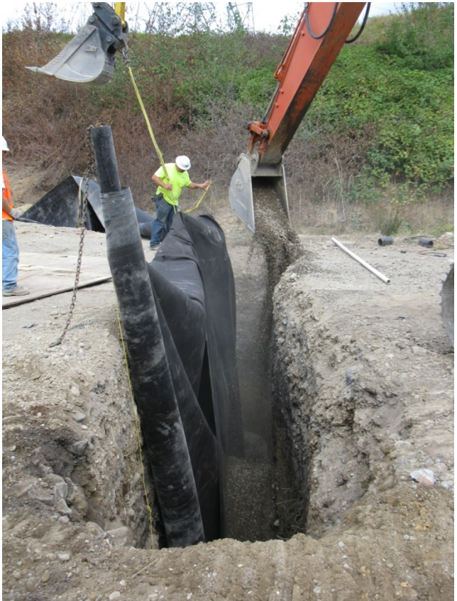
Geotextile/geomembrane "sandwich" getting backfilled
