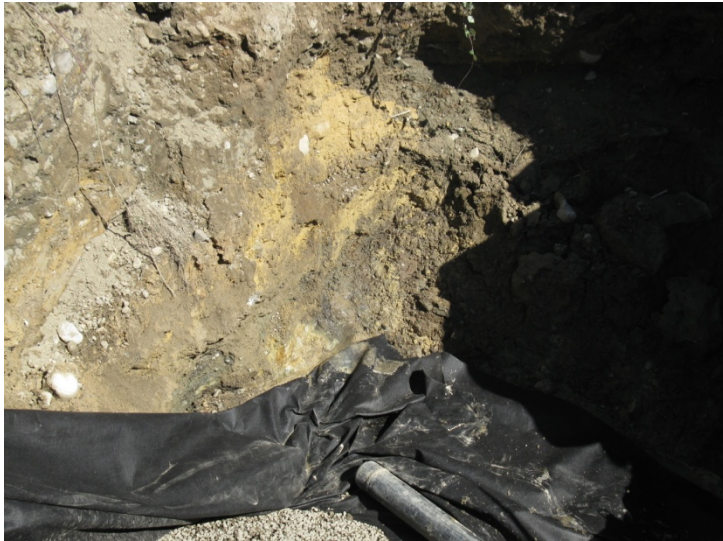
Perforated pipe, 12oz fabric and drainage rock in test pit #2.
