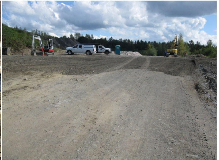
Finished road repair with -2" top course.
