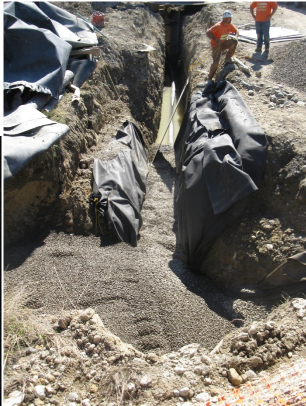
Drainage rock in test pit #2 and trench seep.
