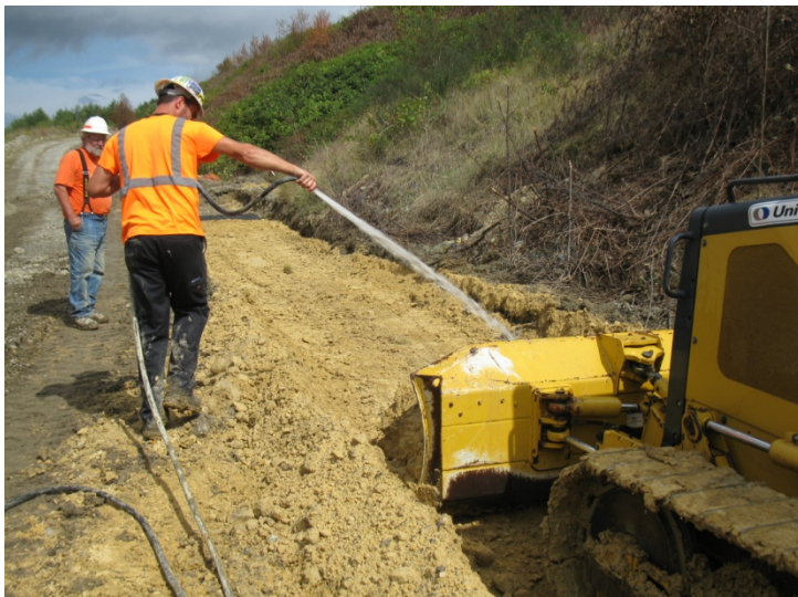
Moisture conditioning soil cap material.
