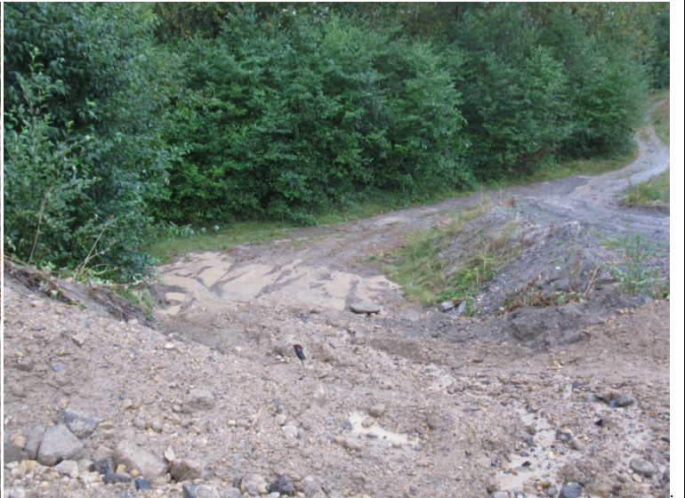
Interceptor trench outfall.
