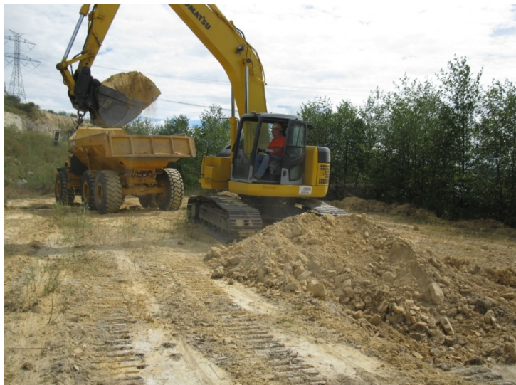
Mine spoils borrow area and low permeable soil cap backfill.
