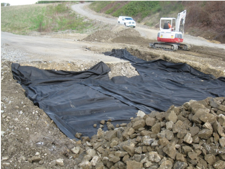
Haul road repair with geotextile fabric and quarry spalls
