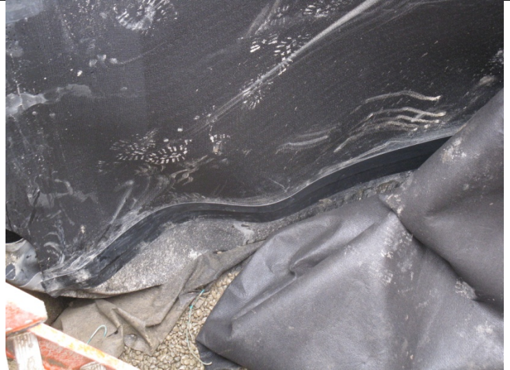
Geomembrane seaming with H-50 tape.
