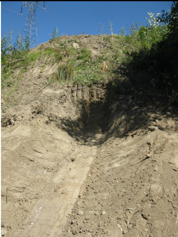
Discharge pipe outlet.
