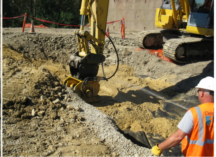
Compaction of low-permeable soil over interceptor trench.
