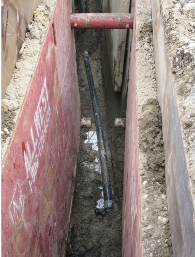
6" HDPE pipe connections with Armor Link couplers.
