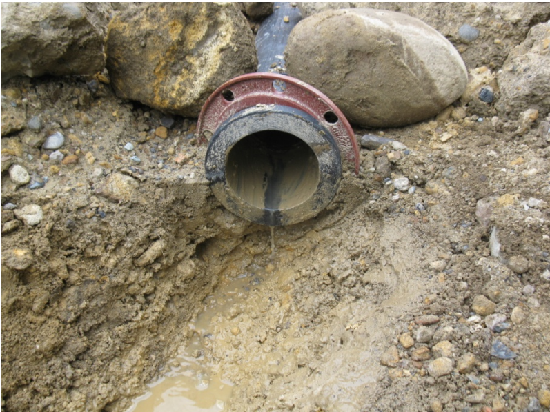
Water flow at interceptor outfall.
