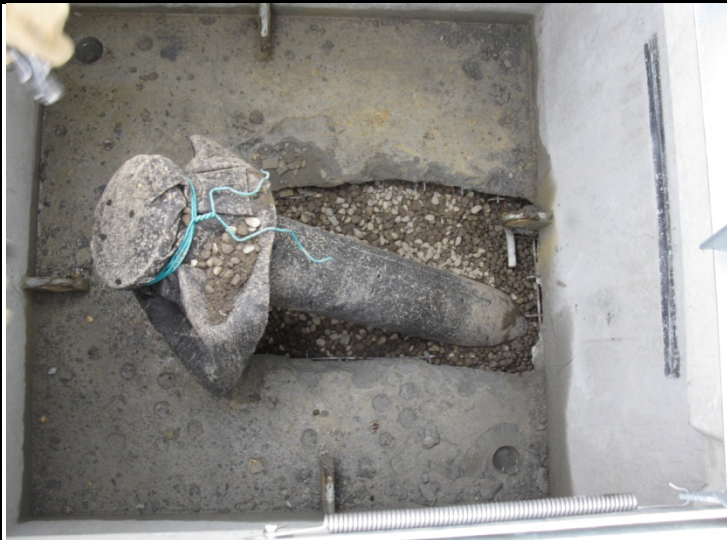
6" pipe penetration into concrete clean out vault.
