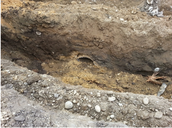
Culvert encountered in test pit 2 drainage trench.
