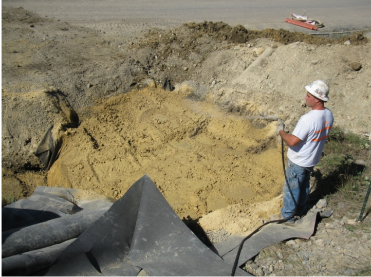
Moisture conditioning of low permeable soil over test pit 2 sump.
