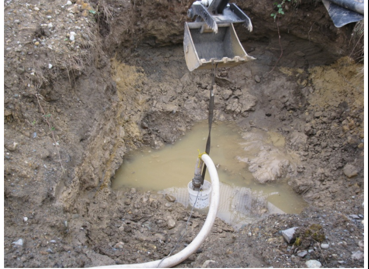
Test pit 2 before clean out.
