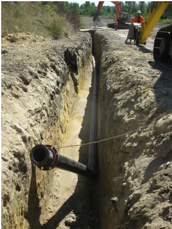
North section of interceptor trench with 6" perforated pipe.
