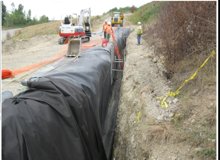
North section of interceptor trench.
