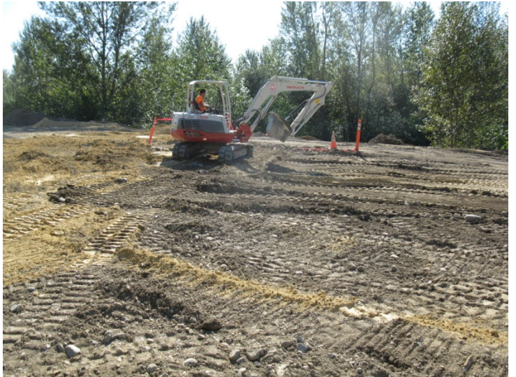
Looking south-west over infiltration trench after backfill.
