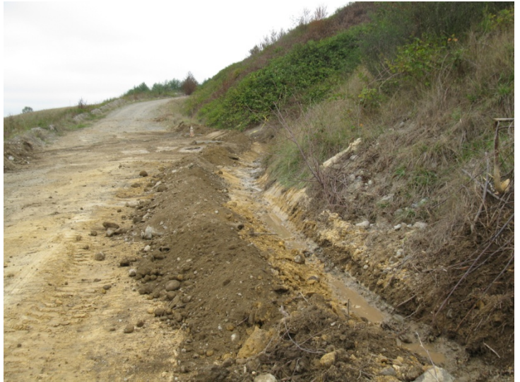
Ditch/berm restoration along upper haul road.
