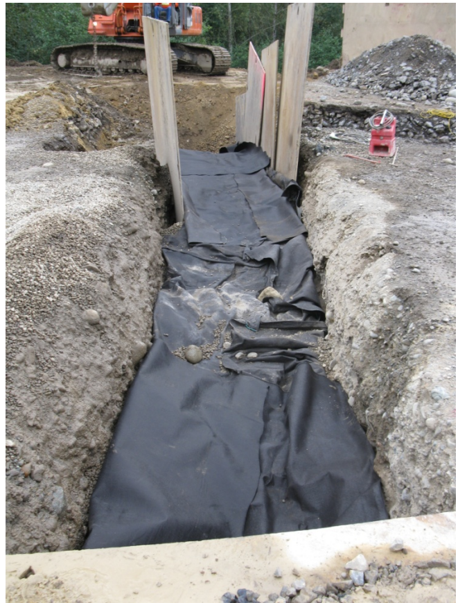
Top of main interceptor trench, drain rock wrapped in 12oz geotextile.
