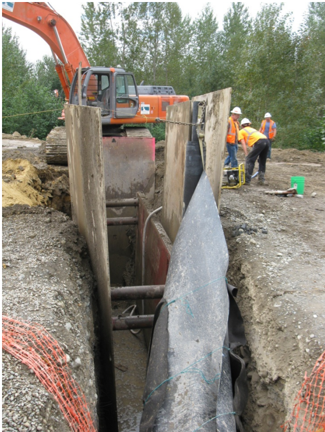
Shoring system in place.
