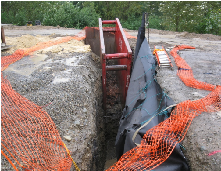
Interceptor trench looking south-west.
