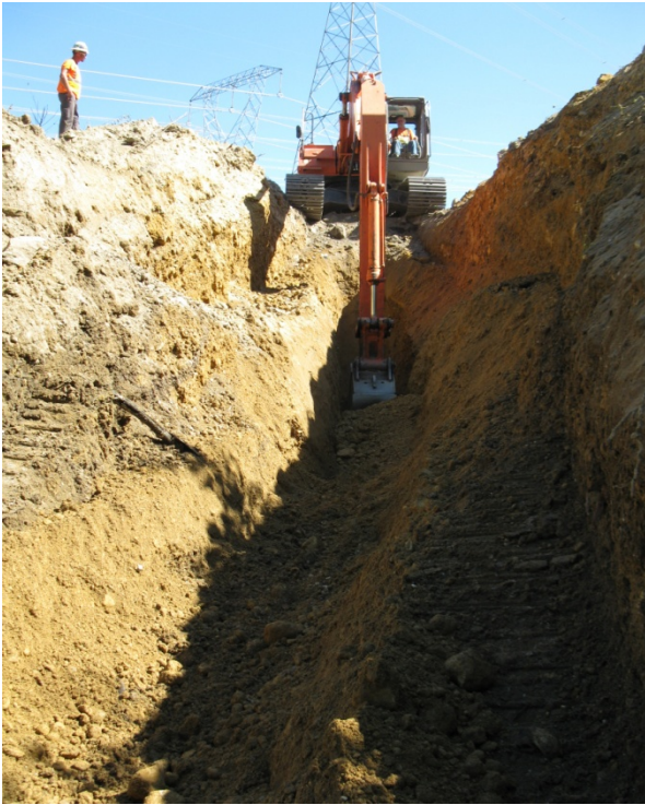
Trench excavation through plug zone looking north-east.
