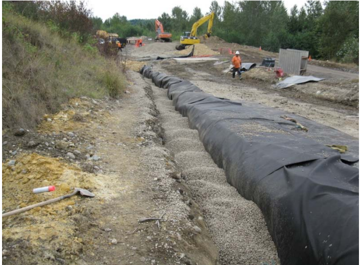
Northern section of trench backfilled with gravel.
