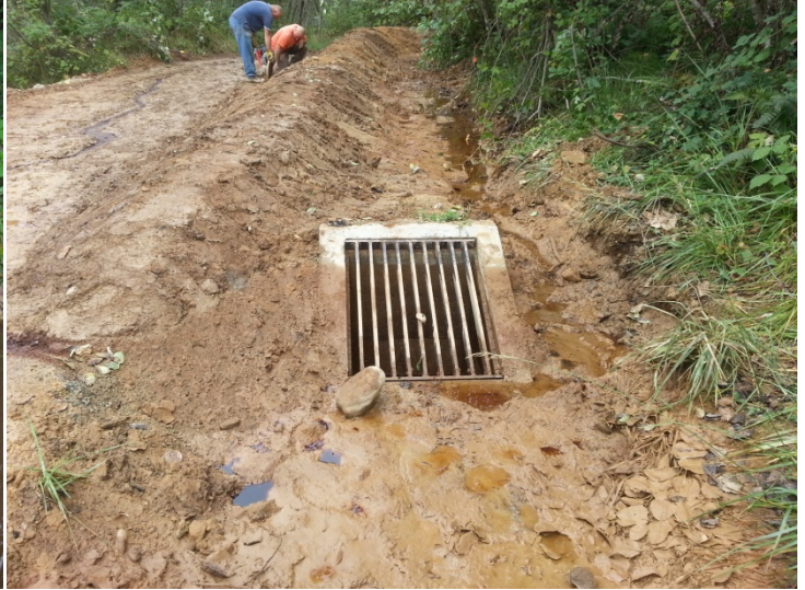
Travertine bench catch basin unplugged after work.
