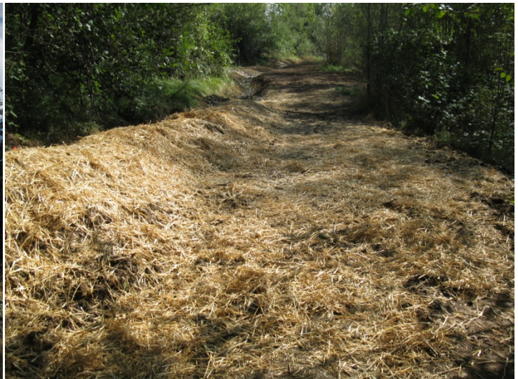
Travertine bench berm and road grass seeded and mulched.
