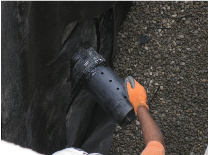
Test pit 2 drainage pipe penetration.
