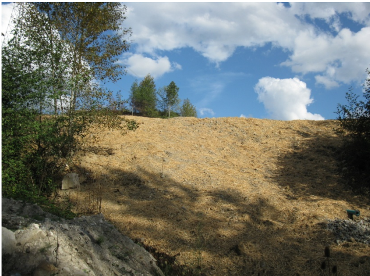
Outfall slope grass seeded and mulched.
