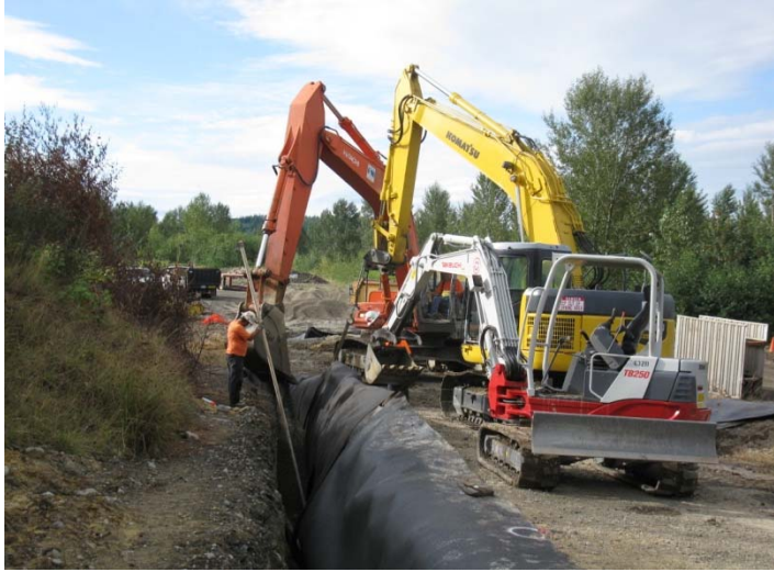
Geomembrane/geotextile installation along north section of trench.
