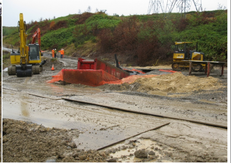
Construction site looking north.
