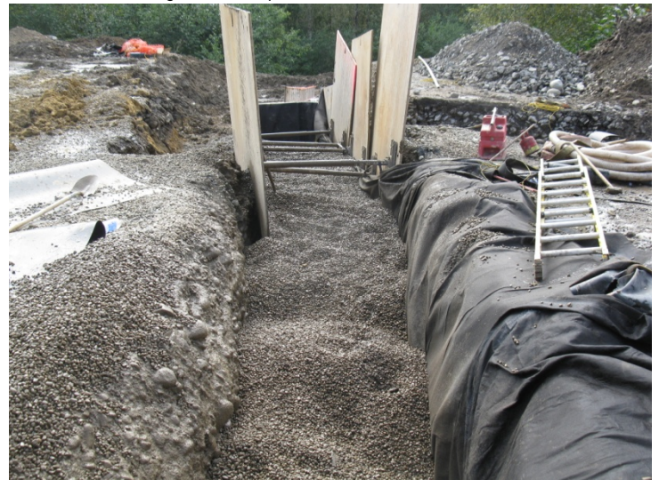
Trench backfilled with -7/8" drain rock.
