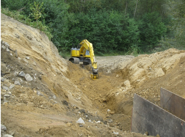
Compaction of fill in pipe plug zone.
