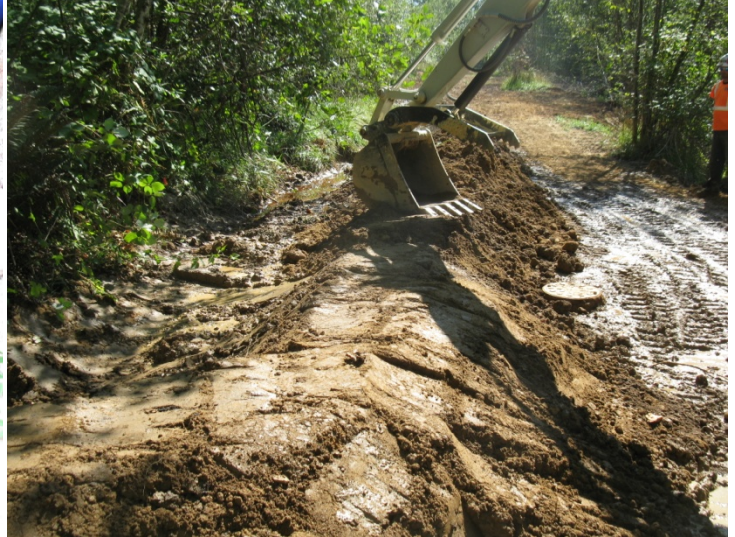
Berm construction on travertine bench.
