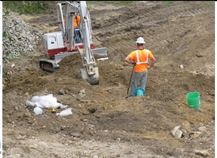
Outfall ditch excavation.
