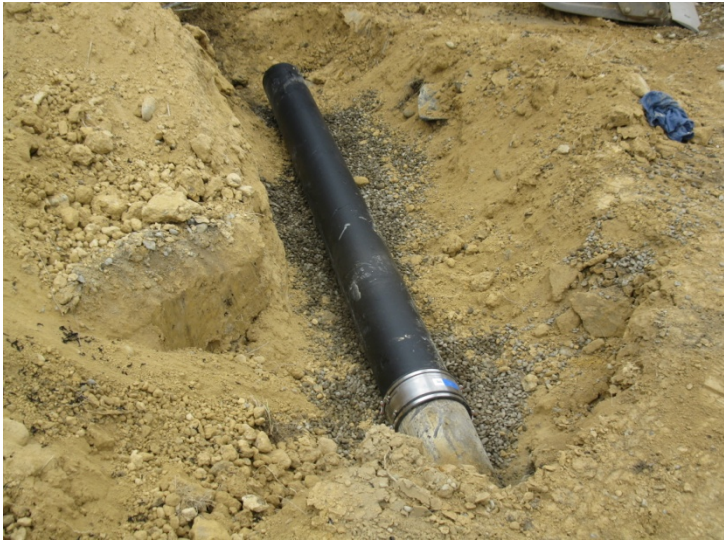
10" HDPE Culvert repair.
