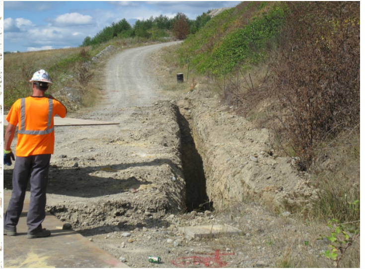
North section of interceptor trench.
