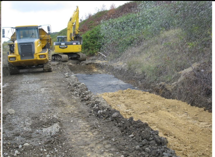
12oz geotextile fabric and loose soil cap looking north.
