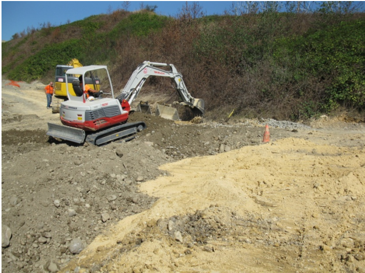
Soil used to backfill top 2' of interceptor trench.
