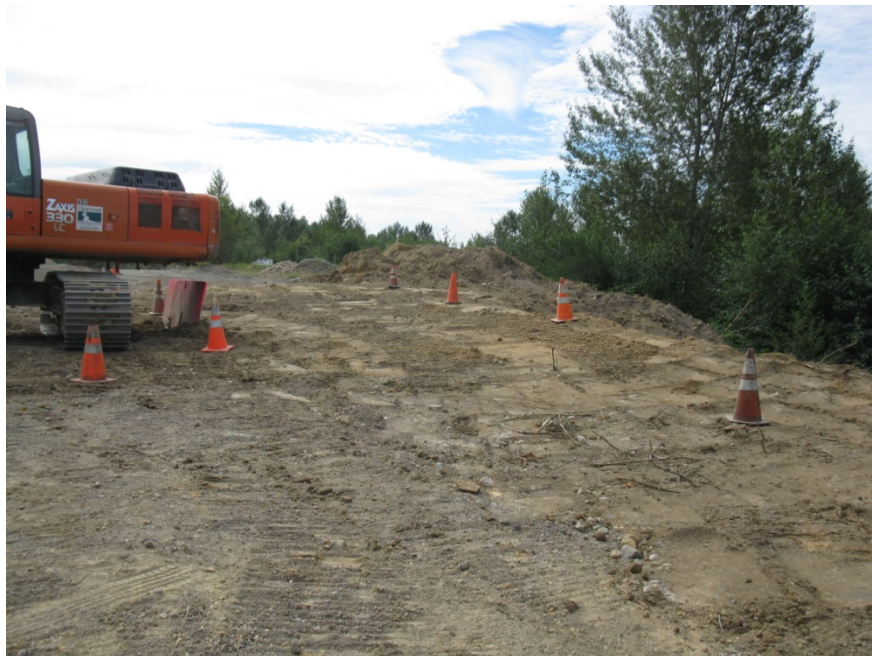
Temporary haul road.
