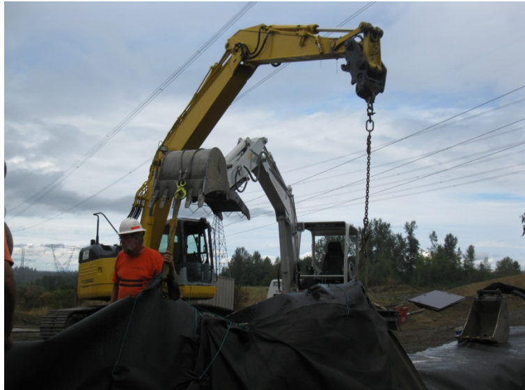
Two excavators pulling wrinkles from geomembrane.
