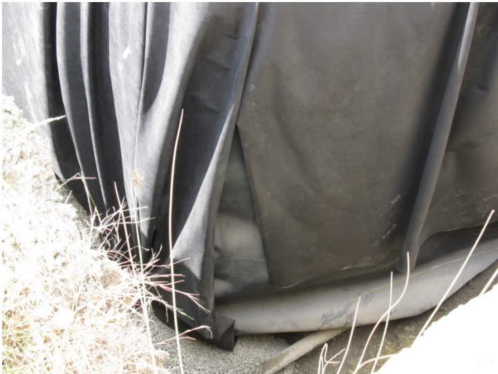
Geomembrane at corner of interceptor trench.
