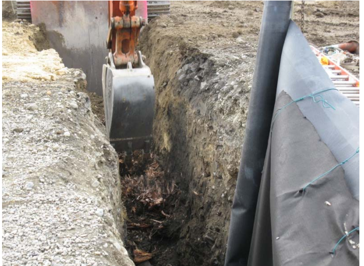
Large stump encountered in trench excavation today.
