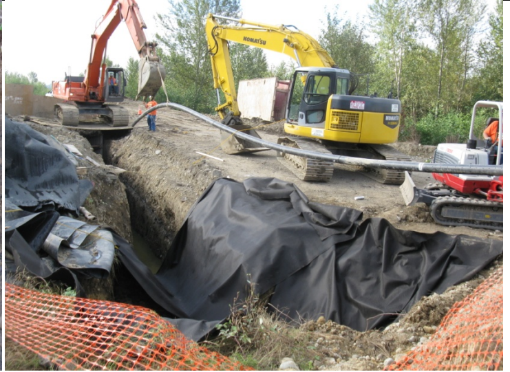
Placement of 6" HDPE pipe into test pit #2 and trench.
