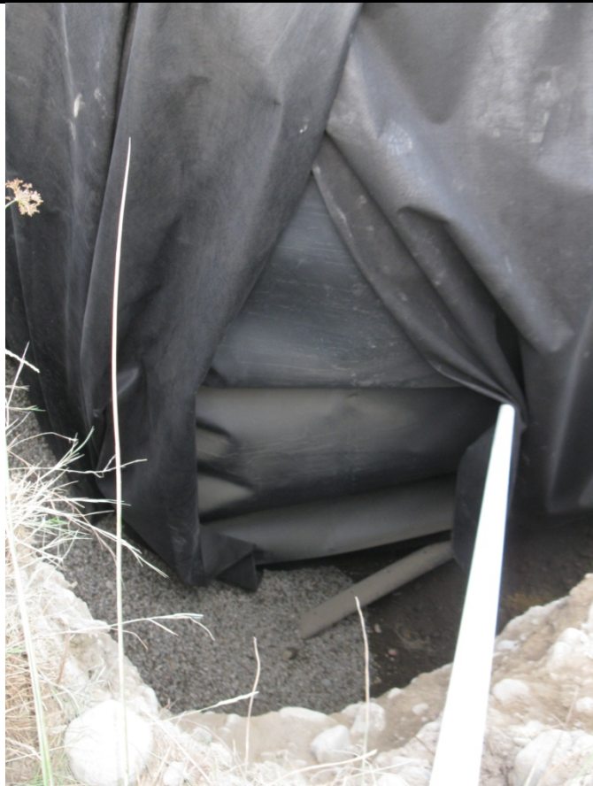
Geomembrane at corner of trench.
