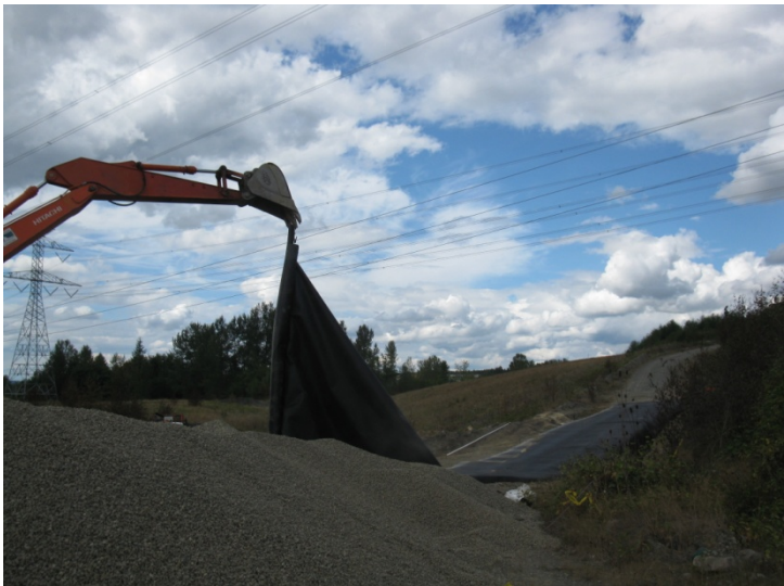
Geomembrane staging along trench.
