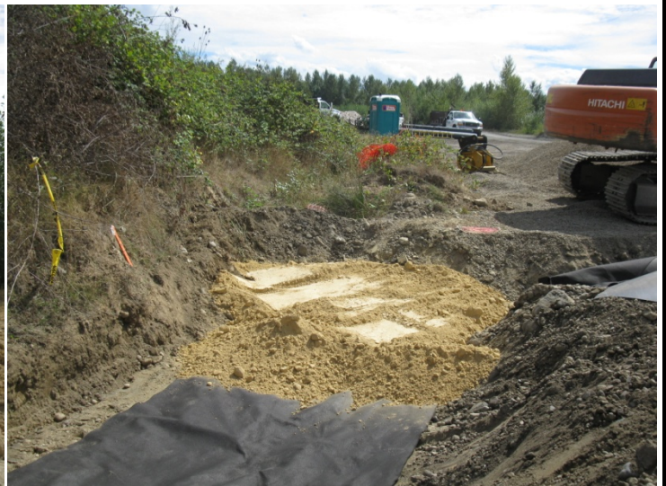
Placement of soil cap for temporary haul road re-route.
