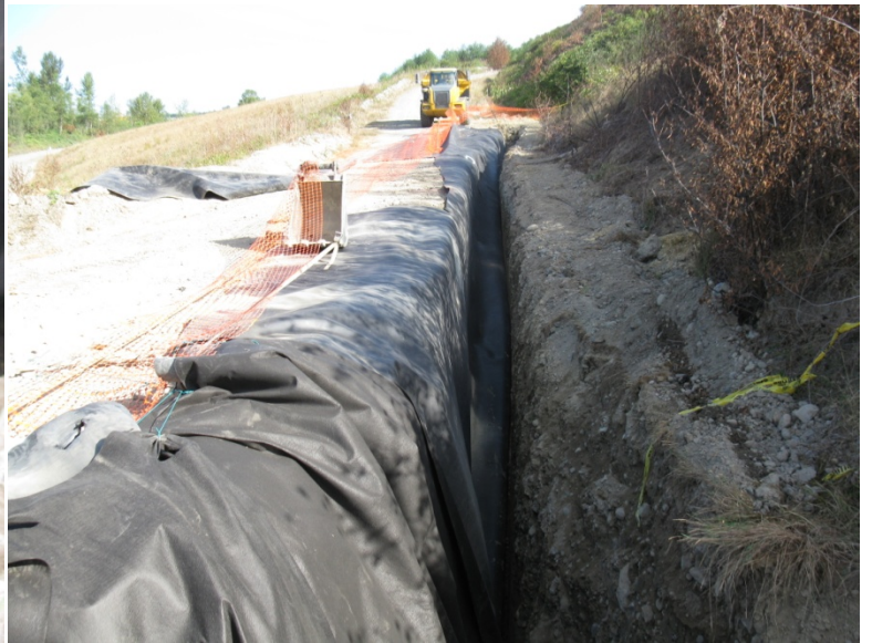
Geomembrane on north section of trench.
