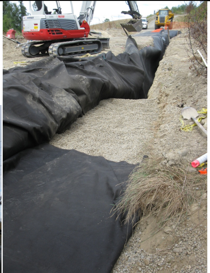
12oz geotextile fabric placed on top of drainage gravel.
