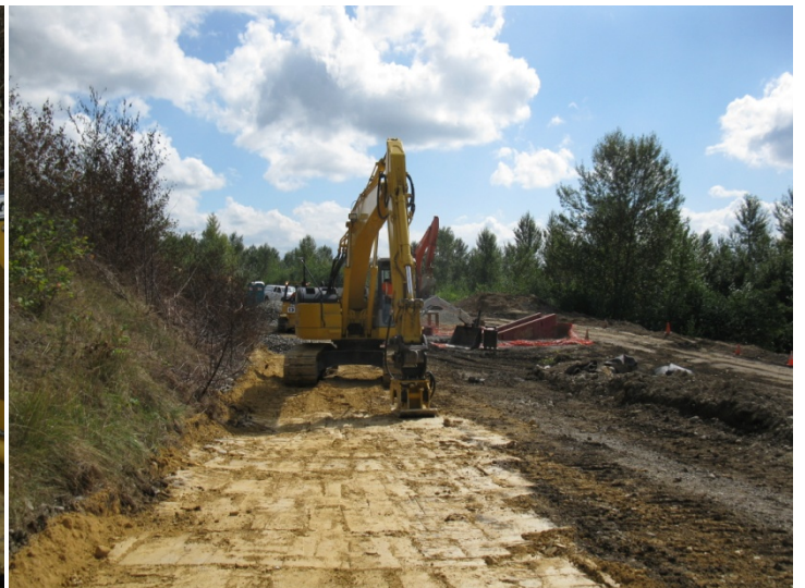
Compaction of soil cap with hoe-pack attachment.
