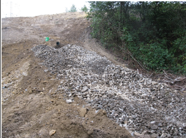
Outfall ditch completed.
