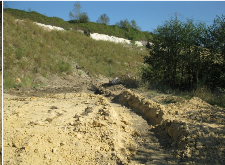
Drainage ditch dug on mine spoils bench.
