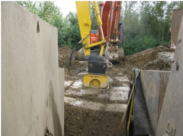
Compaction of plug zone fill.
