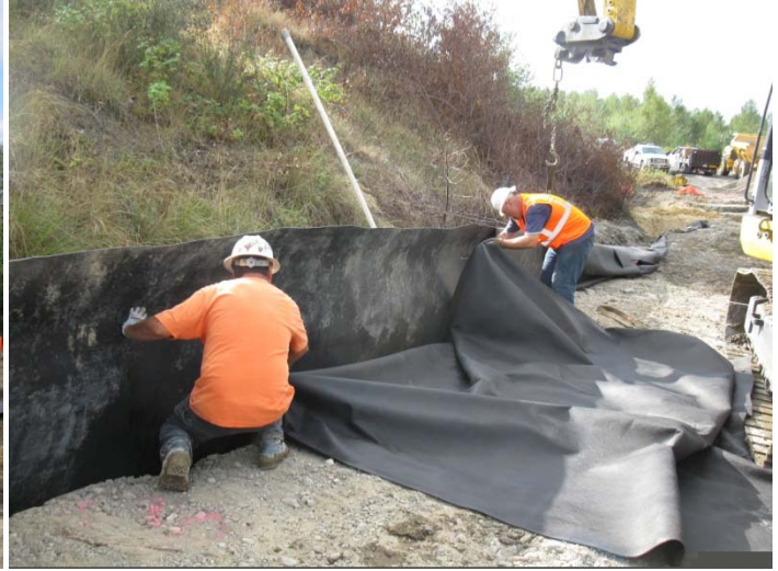
12oz geotextile fabric placed behind geomembrane along trench wall.
