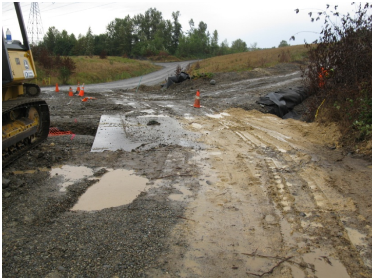
Temporary haul road diversion to the east.
