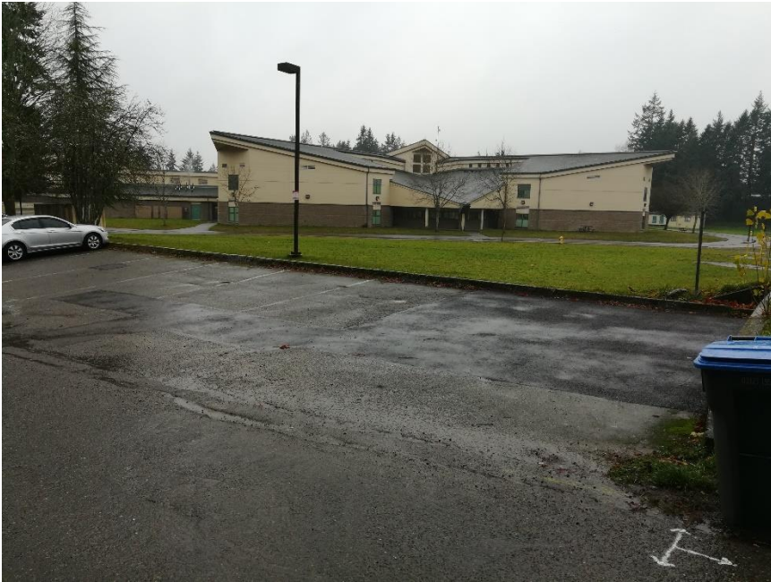
Photo Location 1, 12/11/19 site inspection
