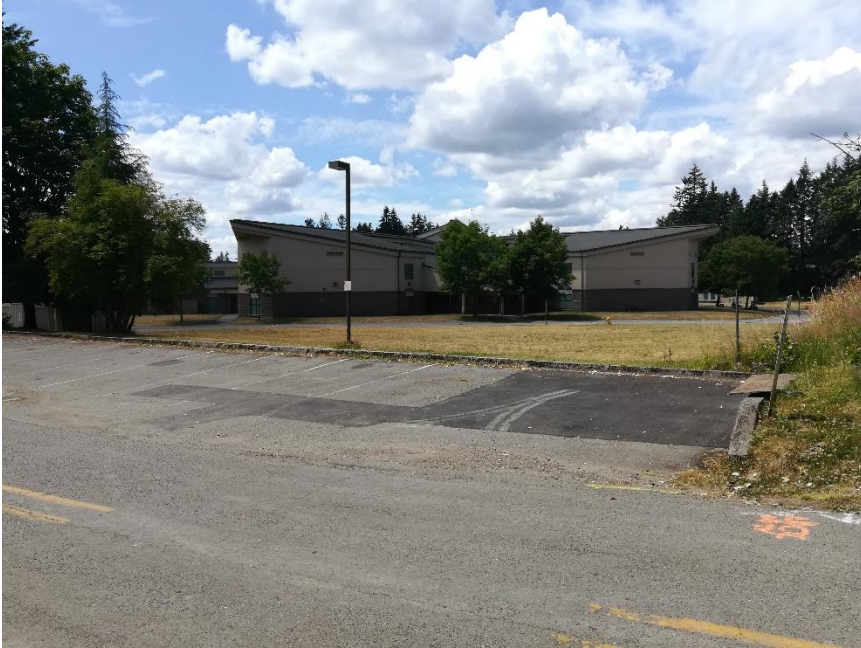
Photo Location 1, 6/25/19 site inspection
