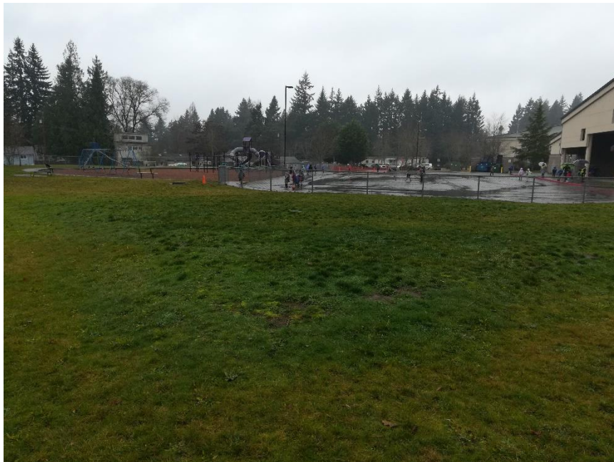
Photo Location 4, 12/11/19 site inspection
