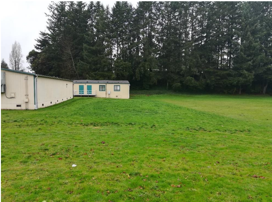
Photo Location 2, 12/11/19 site inspection
