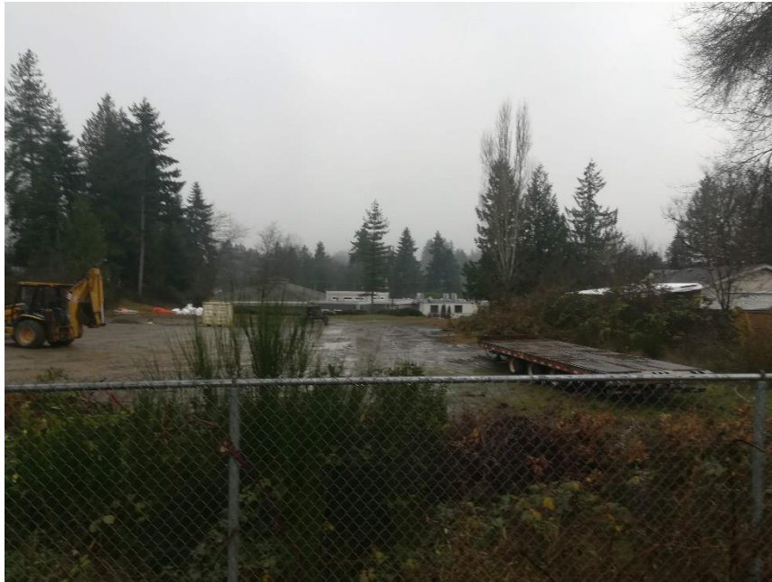
Photo Location 3, 12/11/19 site inspection
