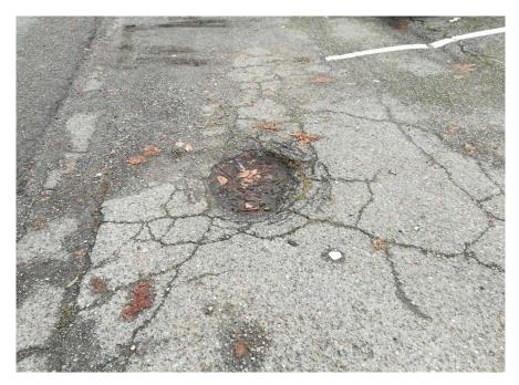
Photograph 3. Photo Location 1 showing pavement deterioration ( $2^{nd}$  view), 12/1/17 site inspection.
