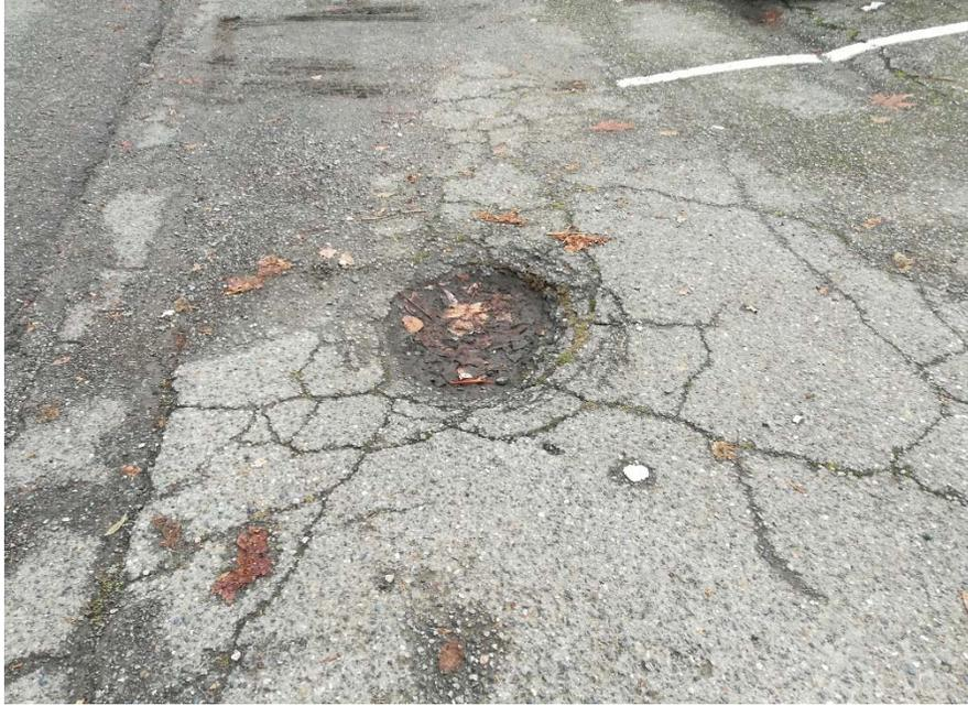
Photograph 3. Photo Location 1 showing pavement deterioration (2<sup>nd</sup> view), 12/1/17 site inspection.
