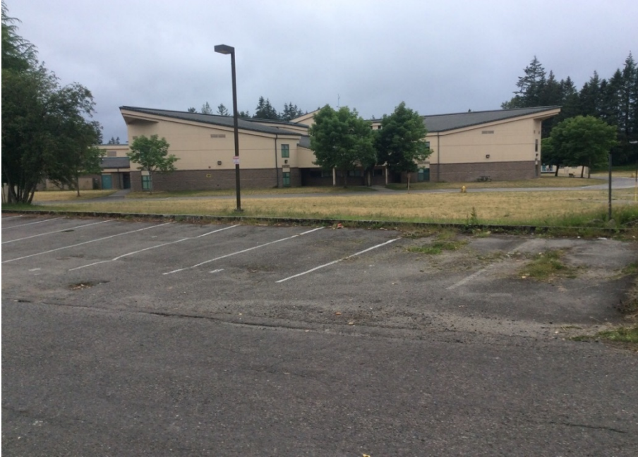
Photo Location 1, 6/22/18 site inspection
