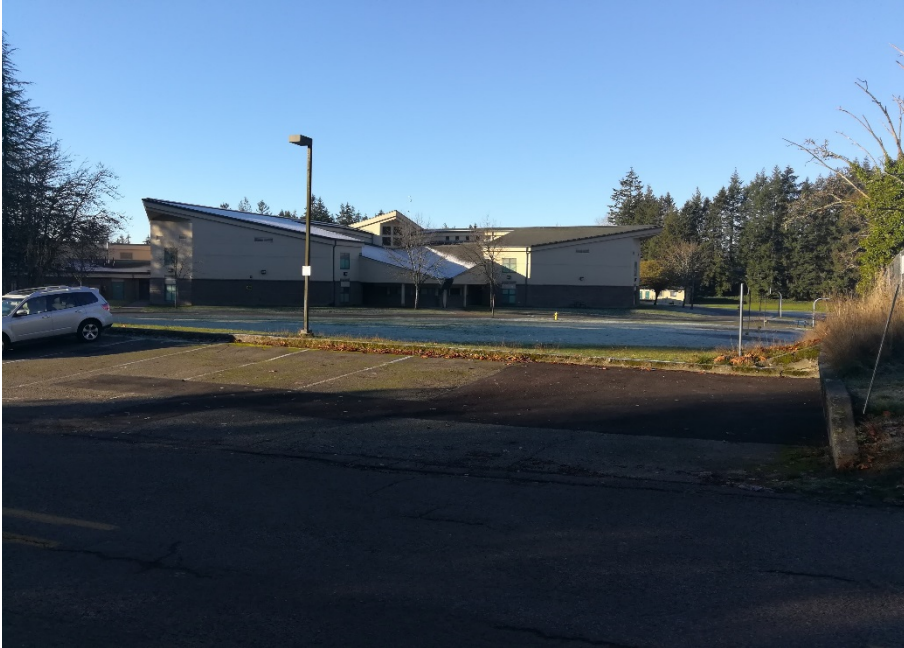
Photo Location 1, 12/4/18 site inspection
