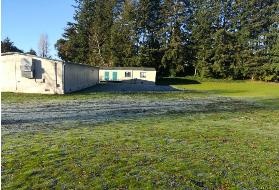
Photo Location 2, 12/4/18 site inspection
