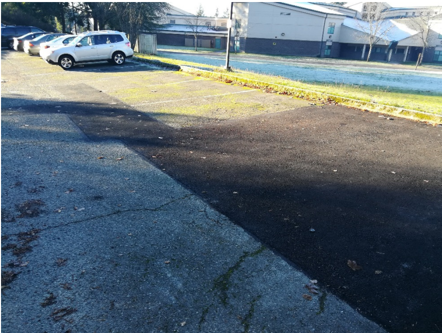
Photo Location 1 showing July 2018 asphalt repair area, 12/4/18 site inspection
