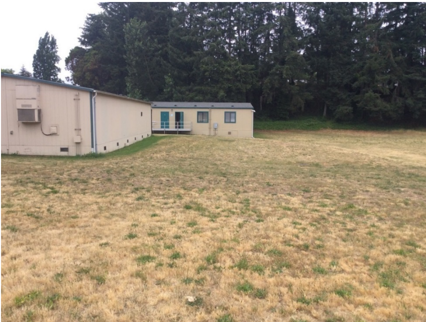
Photo Location 2, 6/22/18 site inspection
