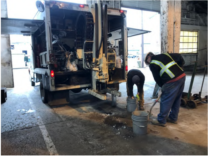
Photograph Six: Drilling of MW9
