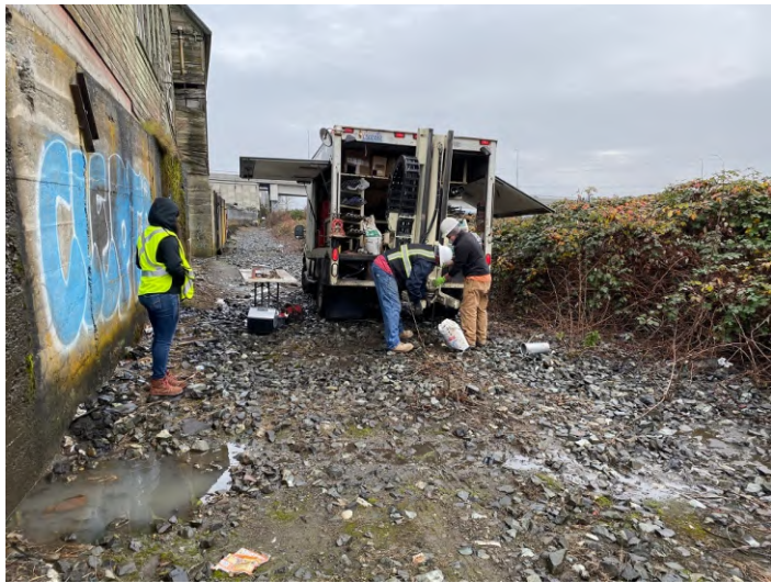
Photograph One: Advancing Boring MW6
