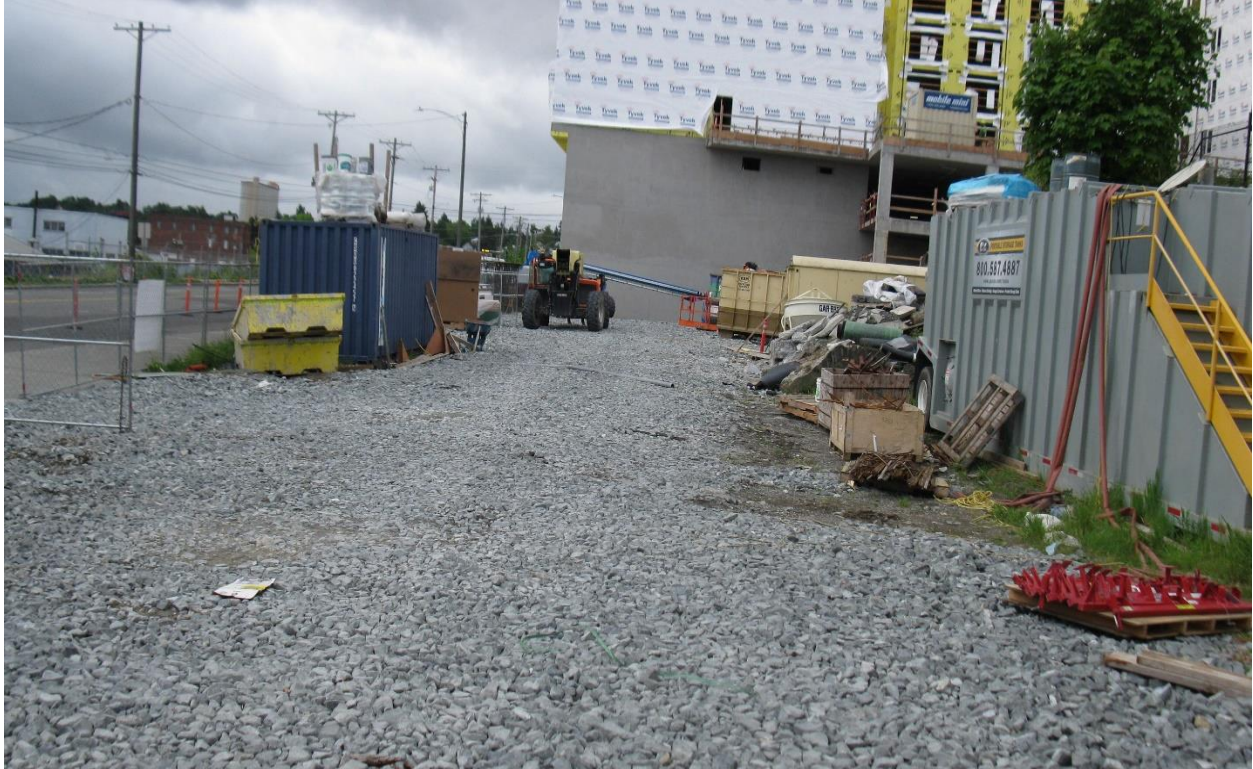
Photo 3: Southern Portion of the Site, Residential Units Construction - From the North
