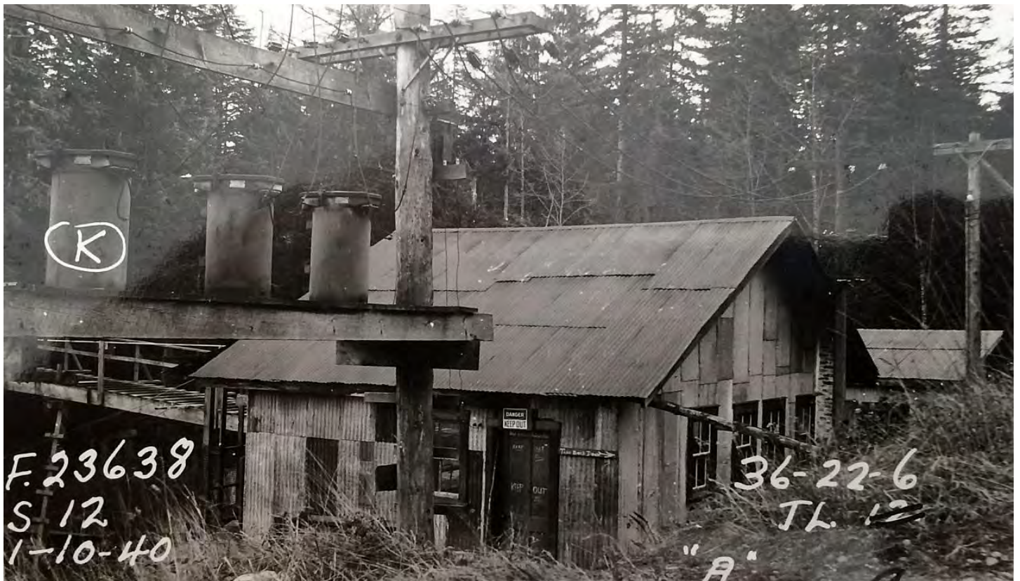
Photo 16-22; Dale Power House-1940 (16 Dale Mines)
