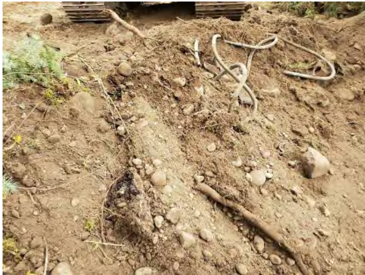
40. Excavation E: Rubber hose and debris encountered during excavation.
