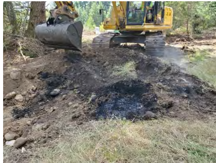
53. Excavation H: Waste oil impacted soils being removed from berm at east end of Excavation H.
