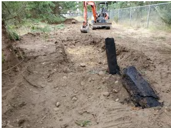
48. Excavation G: Oil stained timbers being removed.
