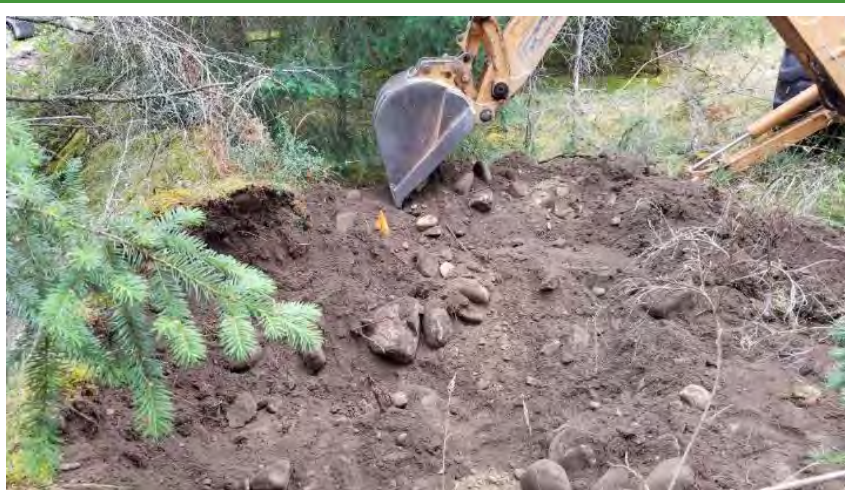
27. Test Pit J – No debris or impacted soils observed.
