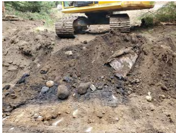
49. Excavation G: Rusted empty 55-gallon drum with oil-stained soils.
