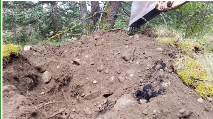
26. Test Pit I with petroleum stained soils.
