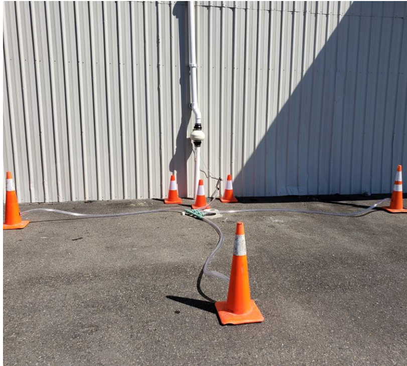
Heated Air Connected to PVC Points and MW-4.
