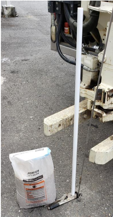
PVC Point Installation.
