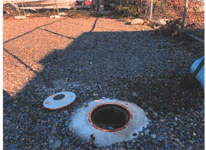
Photo 6 - Replacement Monitoring Well MW4sR
