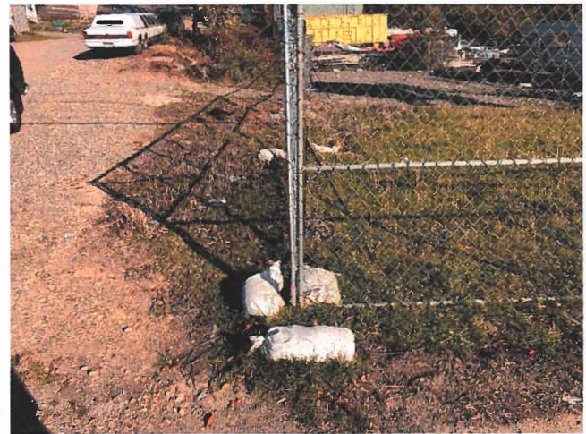
Photo 10 - Southwest Corner of Fencing and Alaska Street
