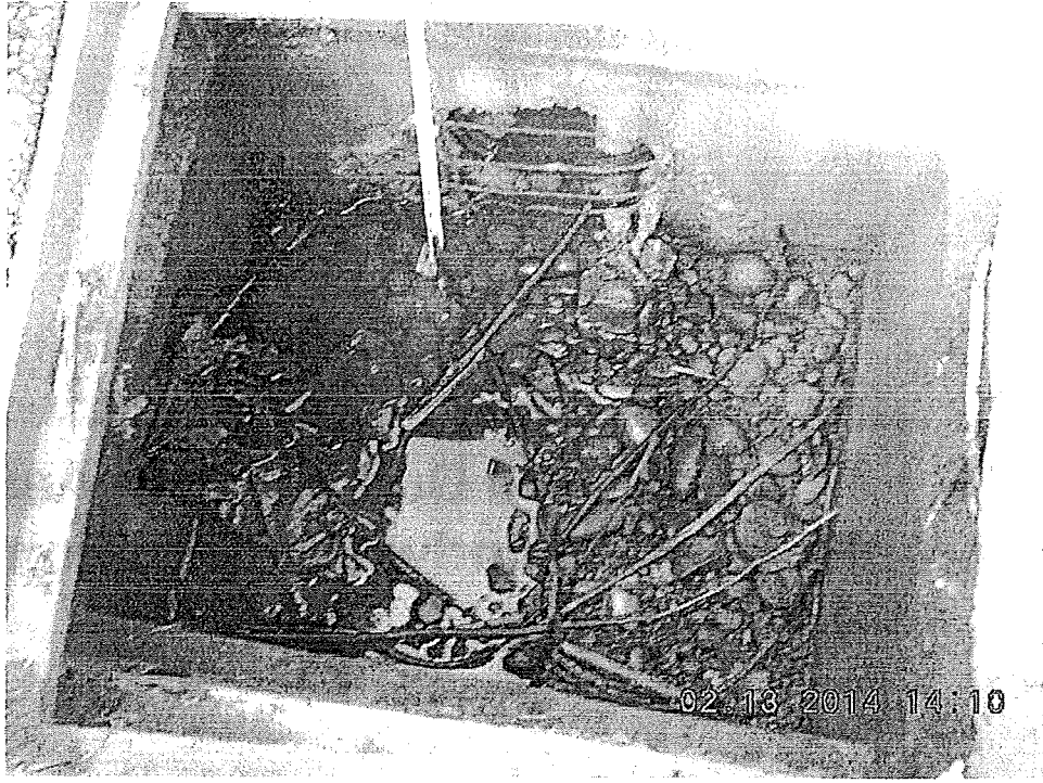
1. South catch basin
