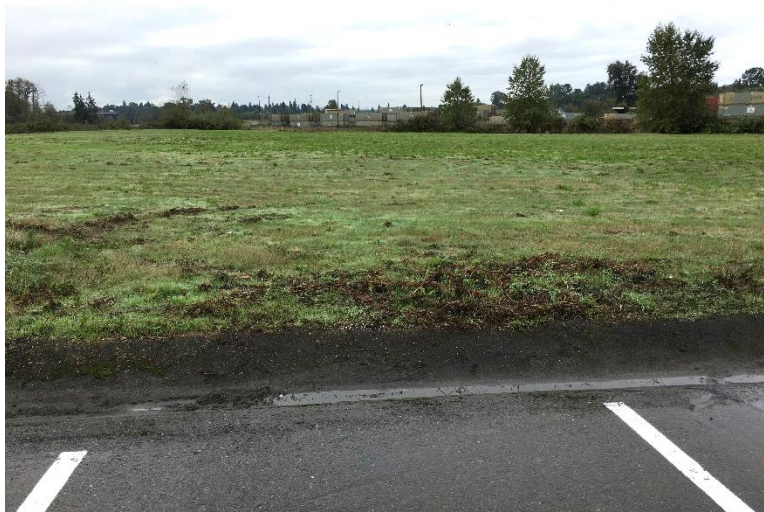
Facing south-southwest from the southern portion of the asphalt cap at the soil cover and the southern drainage ditch.
