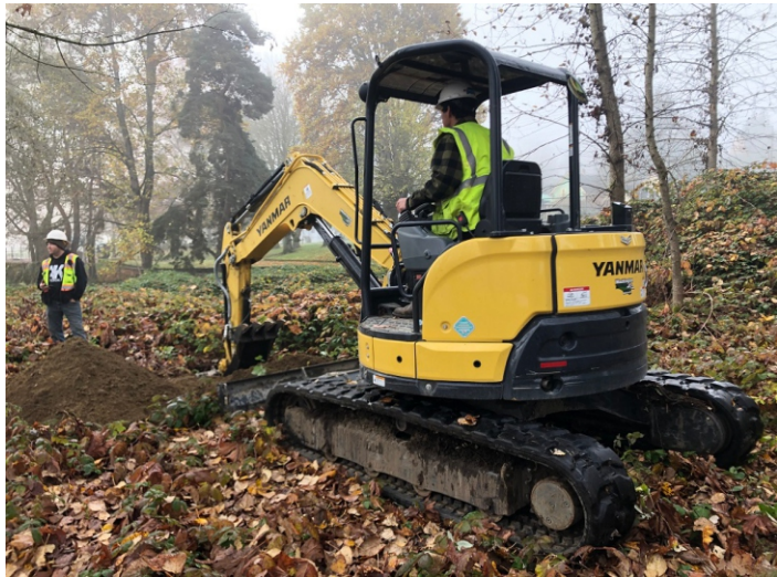
Photograph Five: Excavating Test Pit 2
