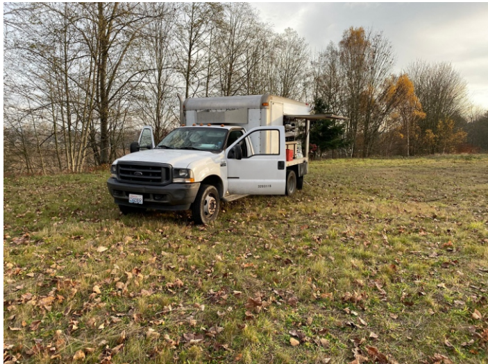
Photograph Three: Advancing Boring B10
