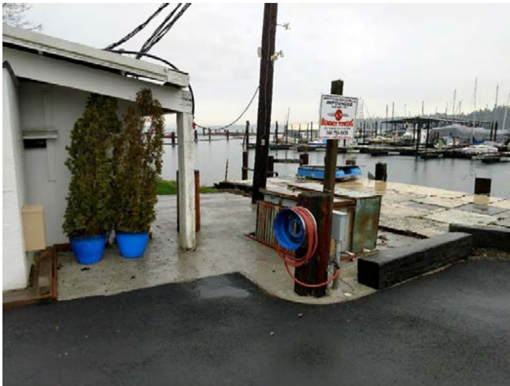
Photograph 11 – View north from the southwest corner of the office structure, showing a portion of the newly installed asphalt paved cap to the south of the structure, and the concrete cap to the east of the structure.
